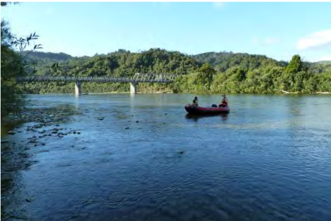
Figure 24 View upstream to x-17 (top) and downstream from x-17 (bottom)
