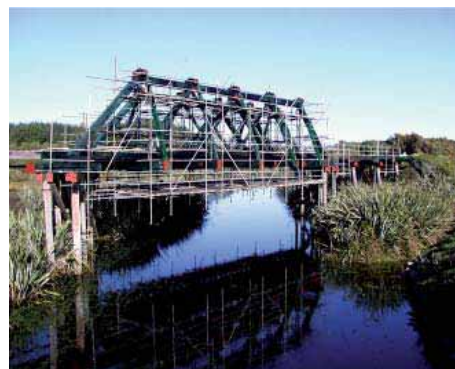
Mahinapua bridge under restoration
