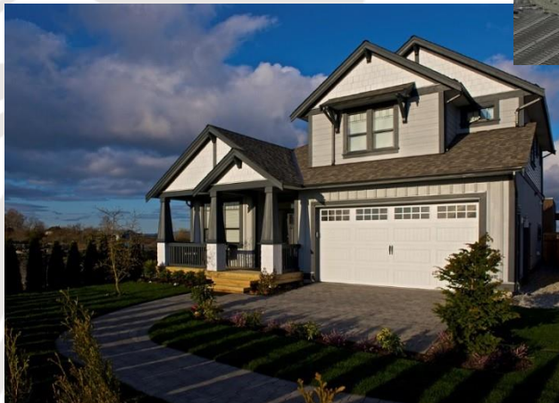
Photo of new leasehold residential unit
