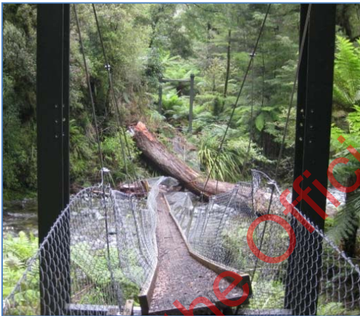
Figure 5.14 Broken main cable and deck structure due to large windfall.
