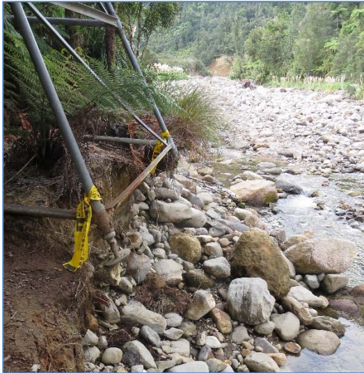
Figure 5.12 Loss of support to NZFS Swingbridge tower footing due to scour.
