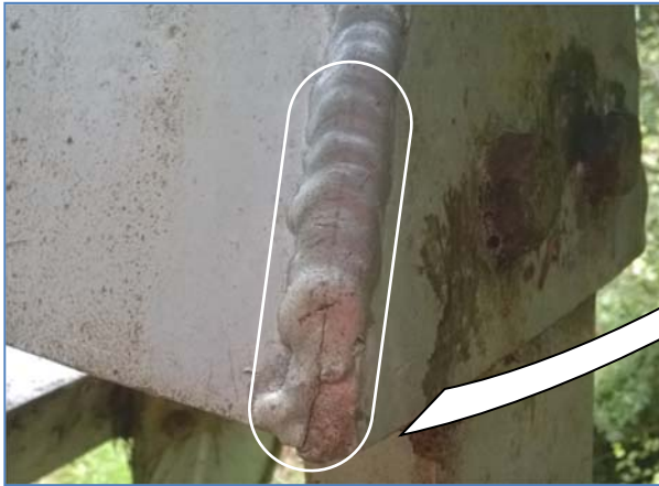
Figure 5.33 Cracked weld, cableway tower
