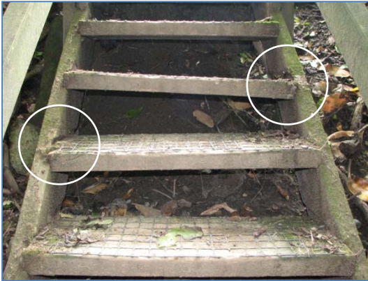
Figure 5.8 Failed tread/stringer connection, common on older staircases.
