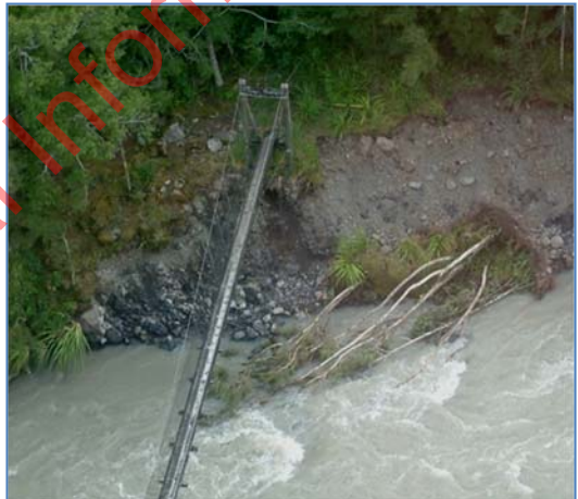
Figure 5.15 Riverbank erosion claims a relatively new suspension bridge.
