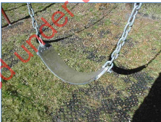
Figure 5.70 Typical swing seat, hanger fixings and chain prone to wear
