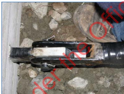
Figure 5.49 Denso Taped cable grips. Should be stripped, torque checked and left exposed.
