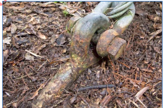
Figure 5.30 Cableway anchor rod & shackle corrosion (acidic soil/leaf-litter/moisture)
