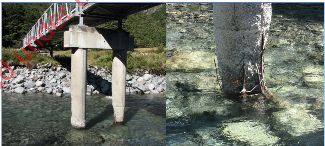
Figure 5.40 Erosion of concrete bridge piers due to impact and abrasion of particles (gravel and rocks) suspended in flood flow.
