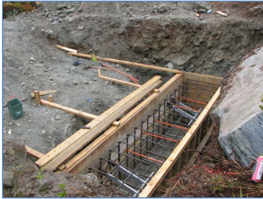
Figure 5.59 Reinforced concrete deadman under construction for suspension bridge main cable anchor.
