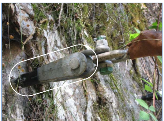
Figure 5.64 Reidbar End-Fittings – Check pin locking wire or 'R-Clip' in place. Check end-fitting not un-winding from rod (it should typically be grouted onto rod or be drilled for locking wire).
