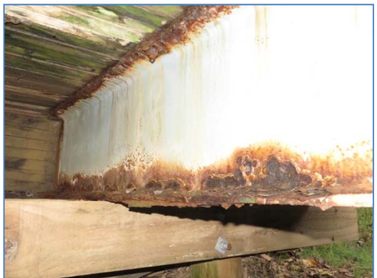
Figure 5.32 Corroded top and bottom flange of vehicle bridge beam
