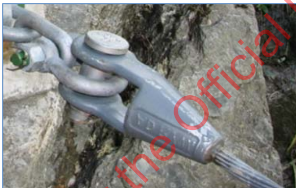
Figures 5.54 – 5.56 Cable termination types
