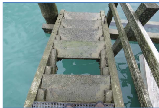
Figure 5.7 Missing stair tread, no anti-slip mesh.
