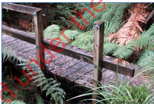
Figure 5.6 Broken/missing barrier rail
