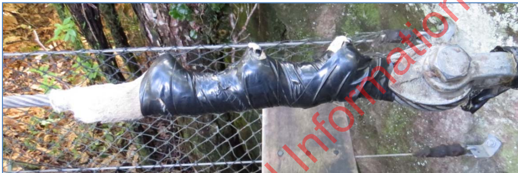
Figure 5.49 Denso Taped cable grips. Should be stripped, torque checked and left exposed.
