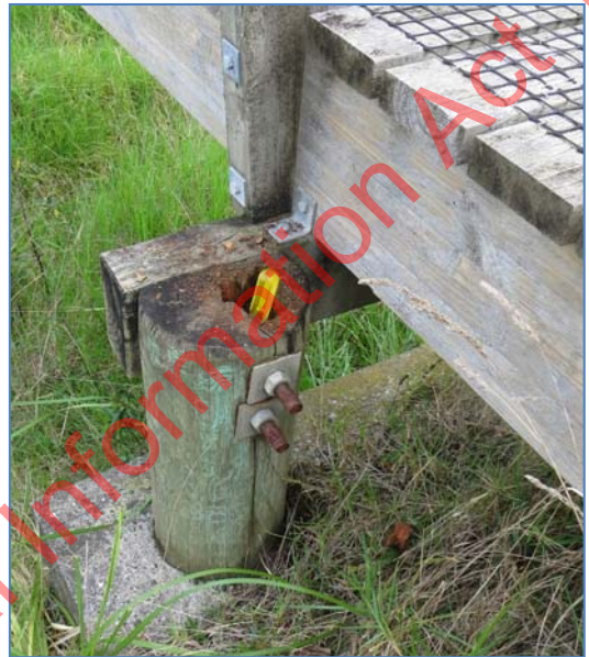
Figure 5.19 Rotten pile
