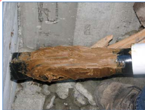
Figure 5.49 Denso Taped cable grips. Should be stripped, torque checked and left exposed.
