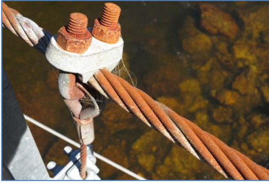
Figure 5.27 Surface corrosion on main cable and wire rope grip U-bolt (hasn't progressed to pitting and section loss yet)
