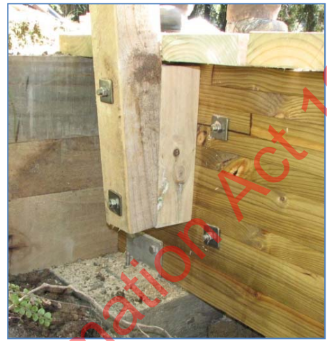
Figure 5.24 New bolted connections can loosen due to timber shrinkage
