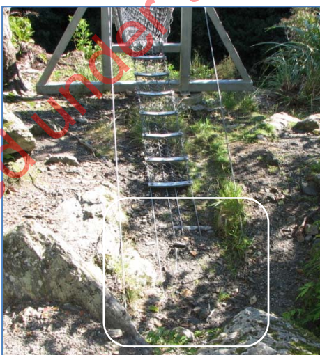
Figure 5.43 Buried NZFS Swingbridge cables and termination hardware
