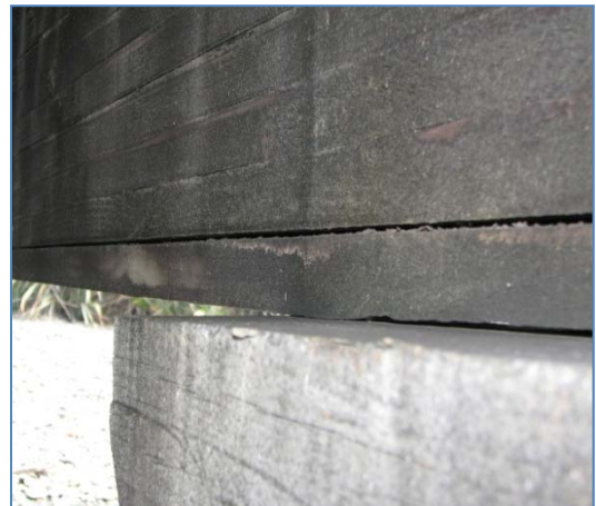
Figure 5.26 Beam strength reduced if entire width of glue-line delaminated
