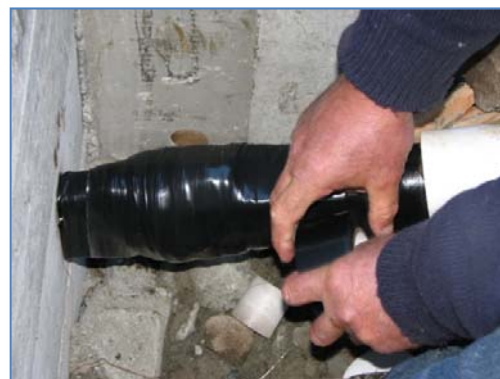
Figures 5.50 – 5.53 Application of the full Denso system (primer paste, fabric tape, PVC overwrap) to an anchor rod component prior to backfilling.
