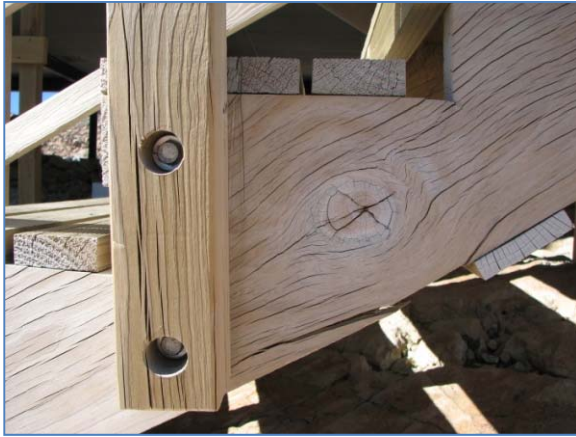
Figure 5.23 Severe drying and splitting of timber in an alpine environment
