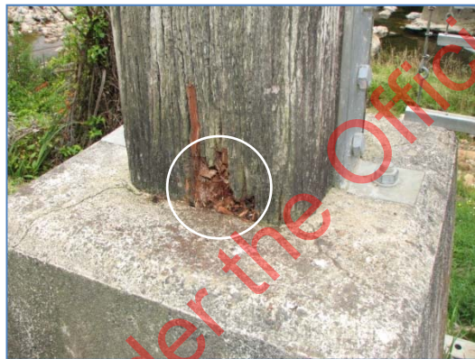
Figure 5.20 Rot at base of suspension bridge tower post
