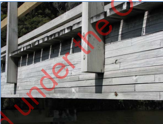
Figure 5.25 Delamination on sunny face of glue laminated timber beam
