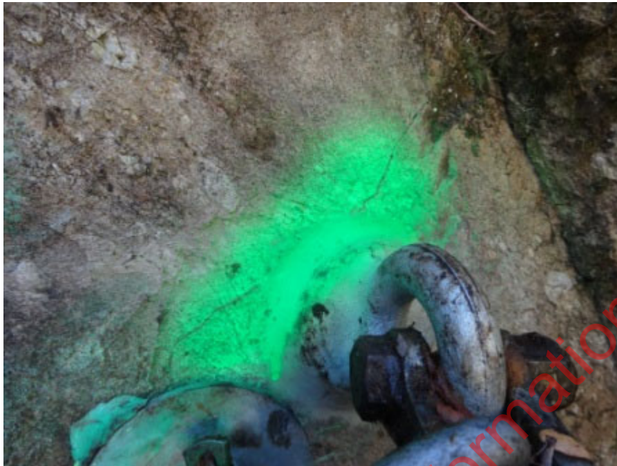
Fig 2: Dazzle paint around rock anchor and existing rock fracture line to check movement. (Note blue tack on old anchor to the left of photo)
