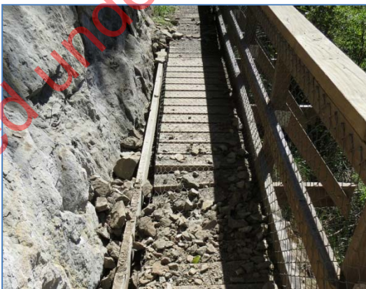
Figure 5.16 Rockfall onto structure. Structure damage less of a concern than the ongoing rockfall hazard to visitors.
