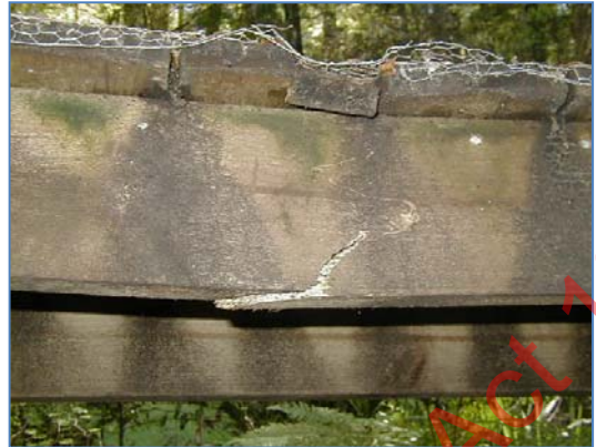
Figure 5.9 Broken sawn timber beam
