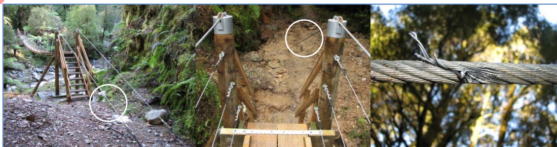
Figure 5.65 Sample photos of damaged swingbridge cable
