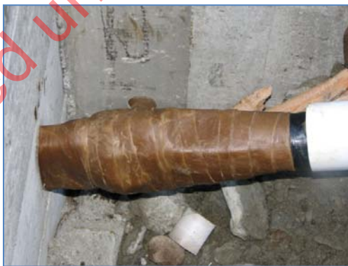
Figures 5.50 – 5.53 Application of the full Denso system (primer paste, fabric tape, PVC overwrap) to an anchor rod component prior to backfilling.
