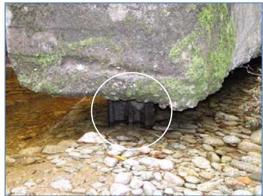
Figure 5.11 There will usually be driven piles under vehicle bridge piers. In this case, because only a short length of the pile is exposed and it's in good condition, no remedial work is required.
