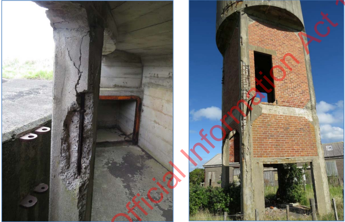
Figures 5.38 & 5.39 Corroded reinforcing steel and spalled cover concrete, historic structures in a marine environment
