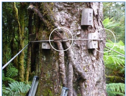
Figure 5.44 3-Wire Crossing hand-cable insufficiently blocked off anchor tree
