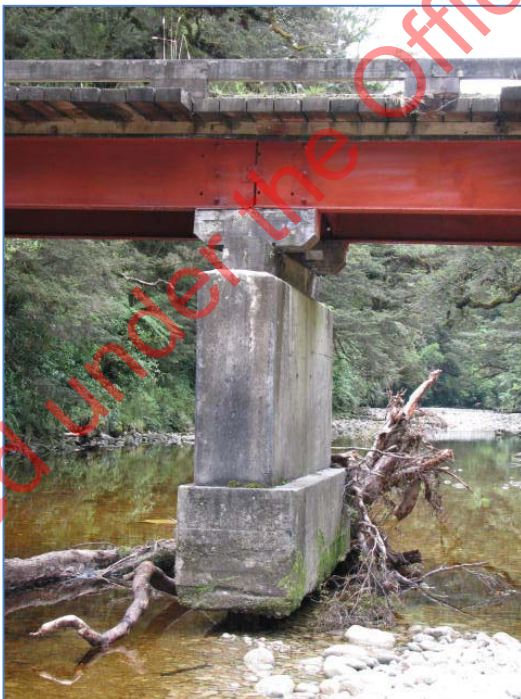
Figure 5.10 Flood debris trapped on a bridge pier can obstruct flow and cause scour – worth removing.
