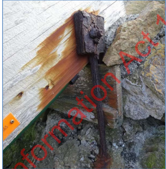
Figure 5.27 Severely corroded stair stringer bracket, marine environment
