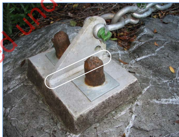
Figure 5.37 Swingbridge rock anchor plate – pay attention to welds – check for cracks.
