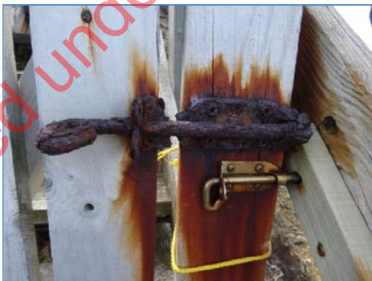
Figure 5.31 Galvanised steel vs. stainless steel in a marine environment
