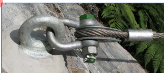
Figure 5.57 Green Pin Standard Bow Shackle with safety bolt
