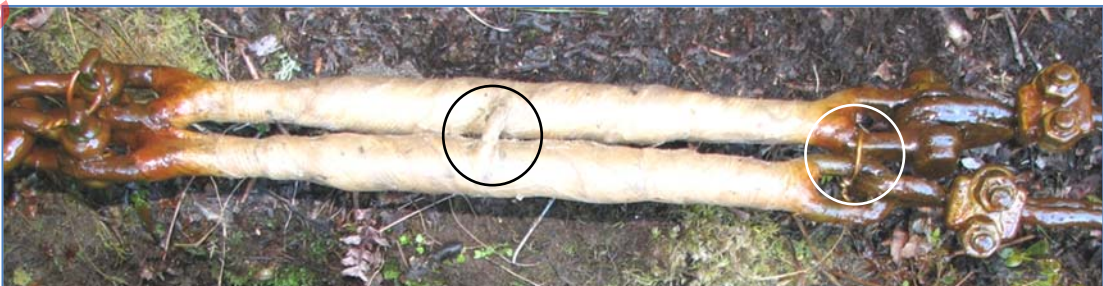
Figure 5.48 Alternative locking wire installation – paired rigging screws wired together. Note installation of Denso Tape for extent of threads only.
