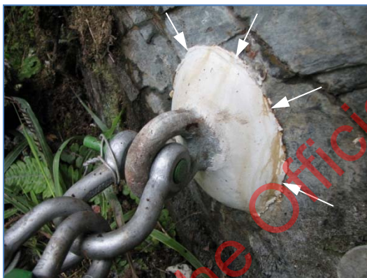
Figure 5.61 Rock Anchor – Check for opening of joint between anchor mortar and rock.
