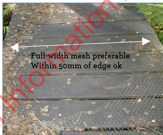
Figure 5.5 Worn anti-slip deck mesh is a common defect and can pose a significant trip or slip hazard.
