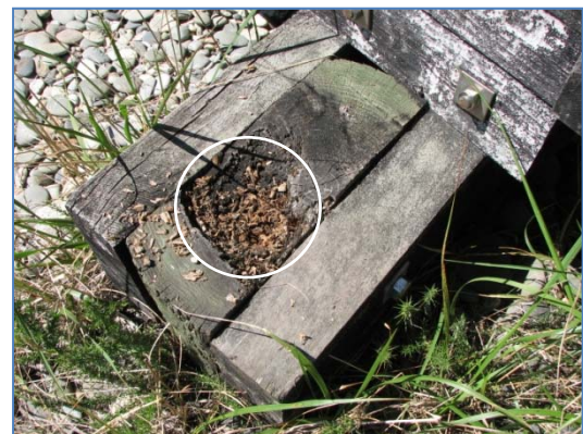
Figure 5.21 Exposed untreated core of pile beginning to rot
