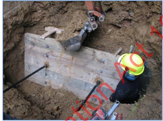
Figure 5.60 Timber deadman under construction for swingbridge main cable anchor.
