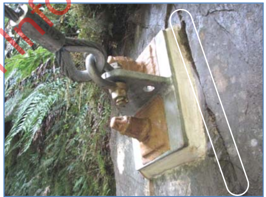
Figure 5.62 Rock Anchor – Check for obvious recent movement of existing cracks around anchor or the development of new cracks.
