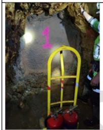
Closed sections are concrete sprayed.
