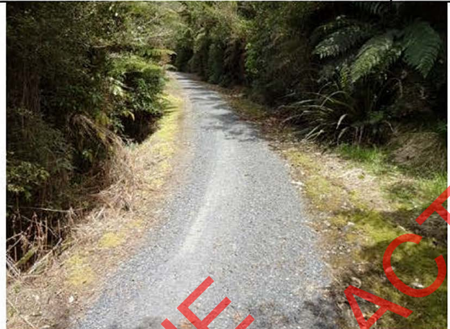
Example where braking impacts are evident.
