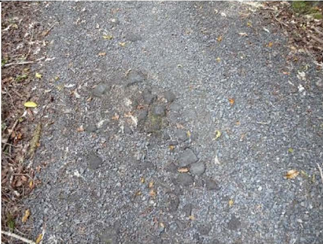
Example of where surfacing top-up is required.
