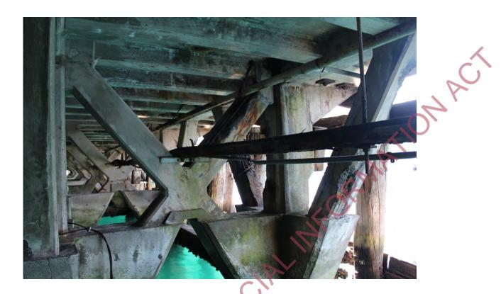
OCEL has undertaken the wharf upgrade design for Waitohi wharf to significantly increase the wharf lateral capacity using 7 separate clusters of 4 raker piles.
