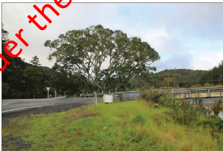
Consider opportunities for the abutments of the old bridge, perhaps as a place for cultural narratives.
