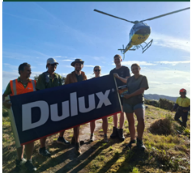
The DOC and Backcountry Trust team restoring Mt Heale Hut on Great Barrier Island / Aotea. Photo: Trevor Cook
