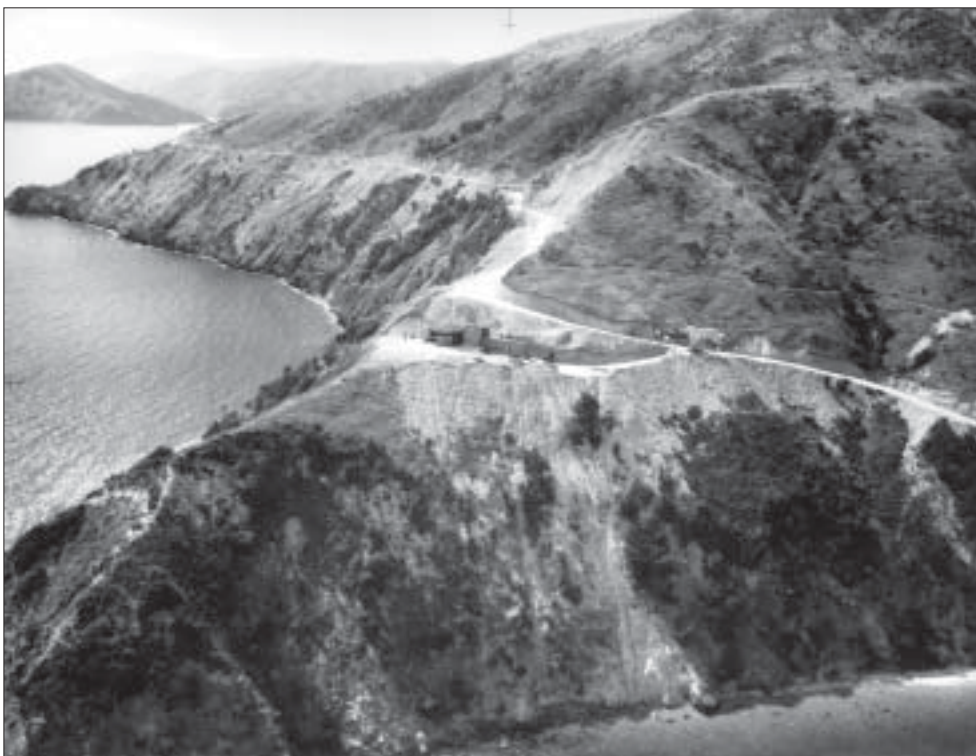
Figure 2. View of first gun emplacement on Blumine Island and road to second emplacement. Photo: NZ Aerial Mapping (F516, taken 1944).
