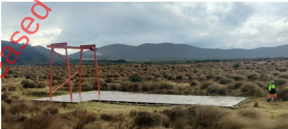
Figure 5 Design of platforms and gantry cranes used in operation
