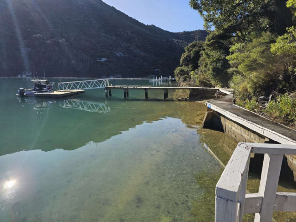
Photo 1: Existing floating jetty, fixed jetty and decking to access boatshed, looking east
