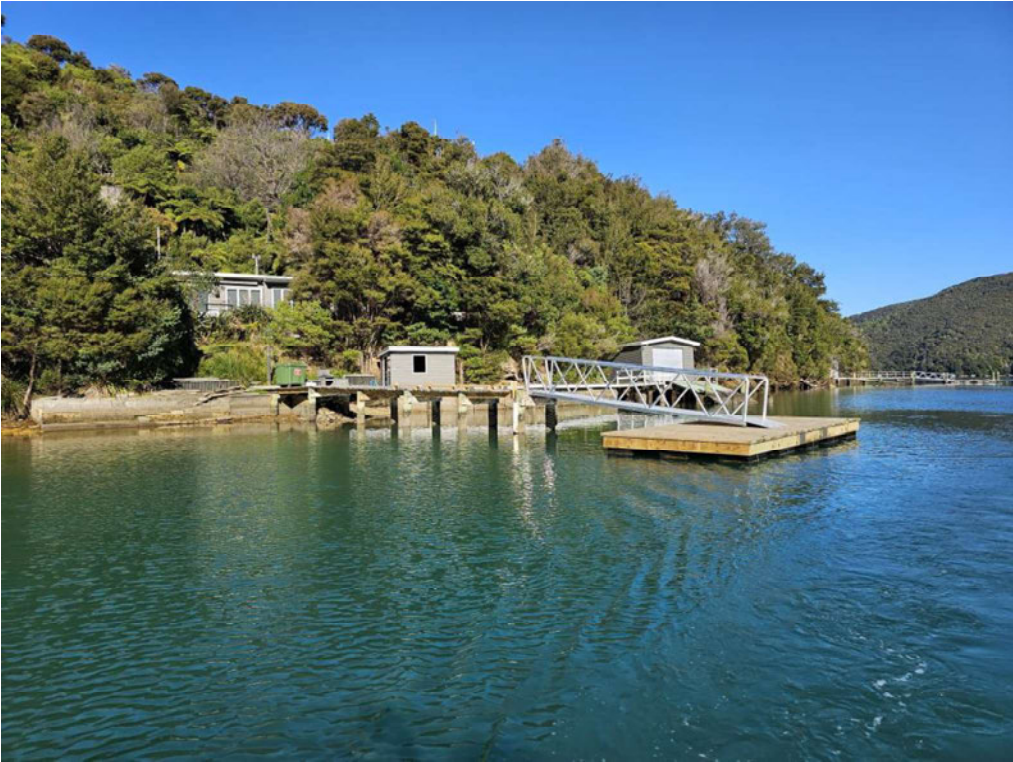
Photo 2: Existing jetty & foreshore structures, dwelling in background, looking west
