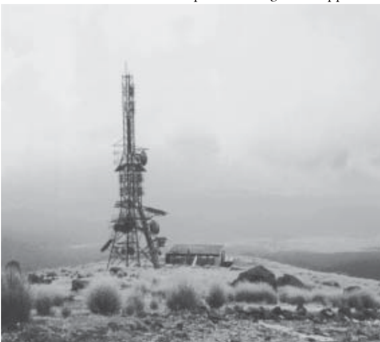
Broadcast Communications Limited's (BCL) Telecommunications Tower on Taburangi. Photo: G Rodley
