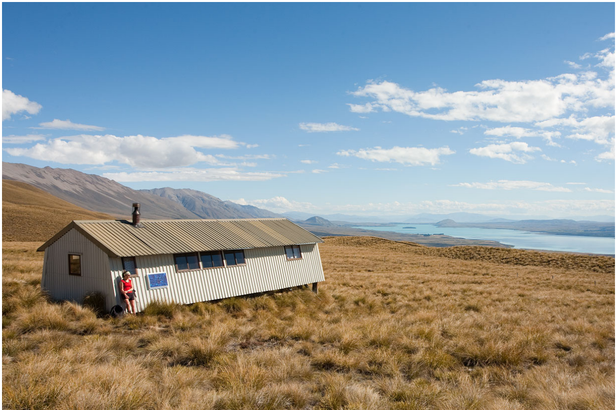
Figure 2: Photo of Rex Simpson Hut from www.alpinerecreation.com , showing the exterior appearance of the hut.
