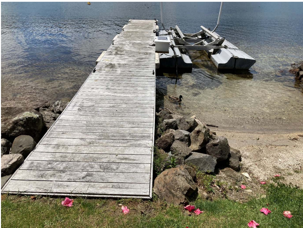
Photo 2 – Existing Jetty G57 and Boat Lifter
