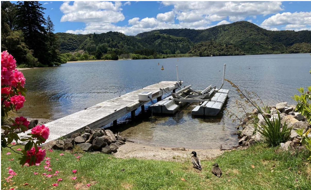
Photo 1 – Existing Jetty G57 and Boat Lifter
