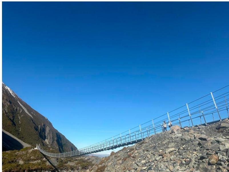
Hooker Valley Bridge no.2. Photo: DOC
