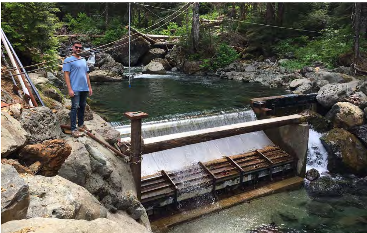
Figure 1 - Example of a Coanda weir
