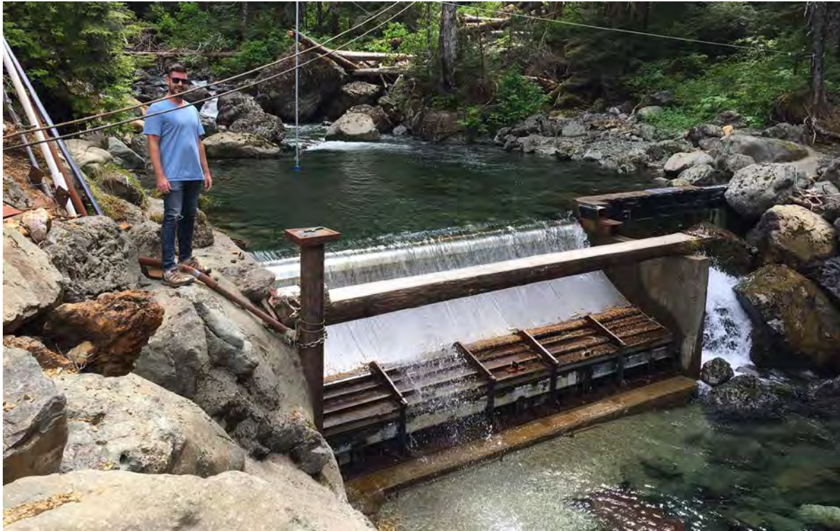
Figure 5 – Example of a Coanda style intake
