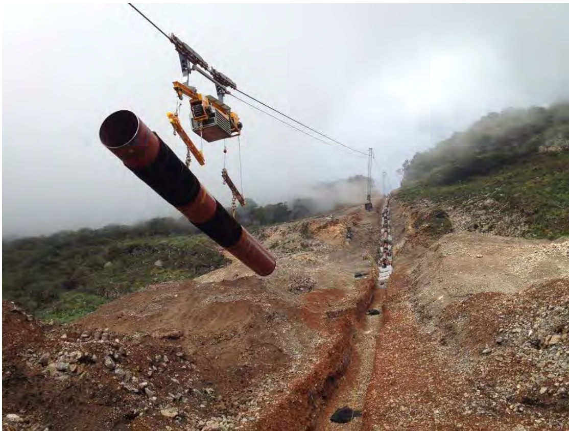
Figure 12 – Example of cableway used for penstock construction
