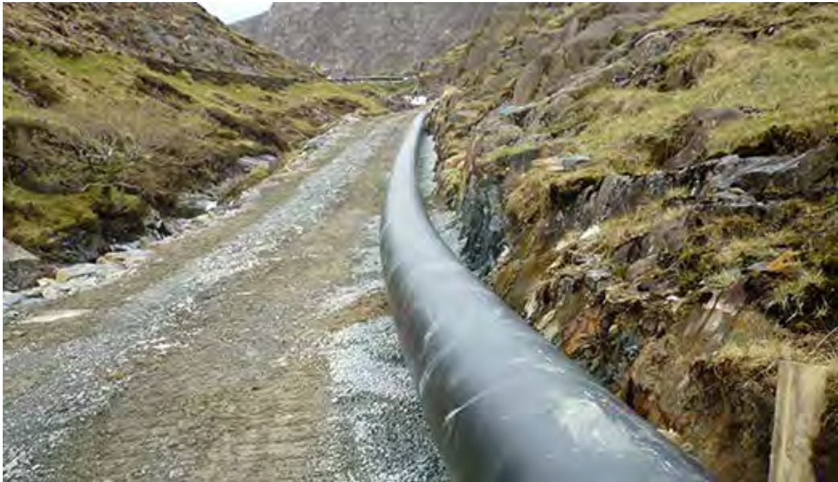
Figure 8 - Example of HDPE penstock alignment
