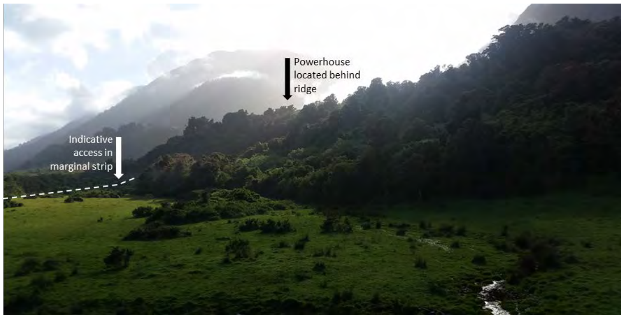
Figure 33 – View from south side of McCulloughs Creek Bridge on Highway 6 showing view obscured by forest cover.
