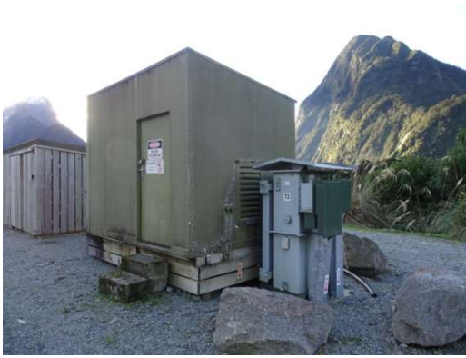
Switching hut and transformer that the BESS will connect to shown on right
