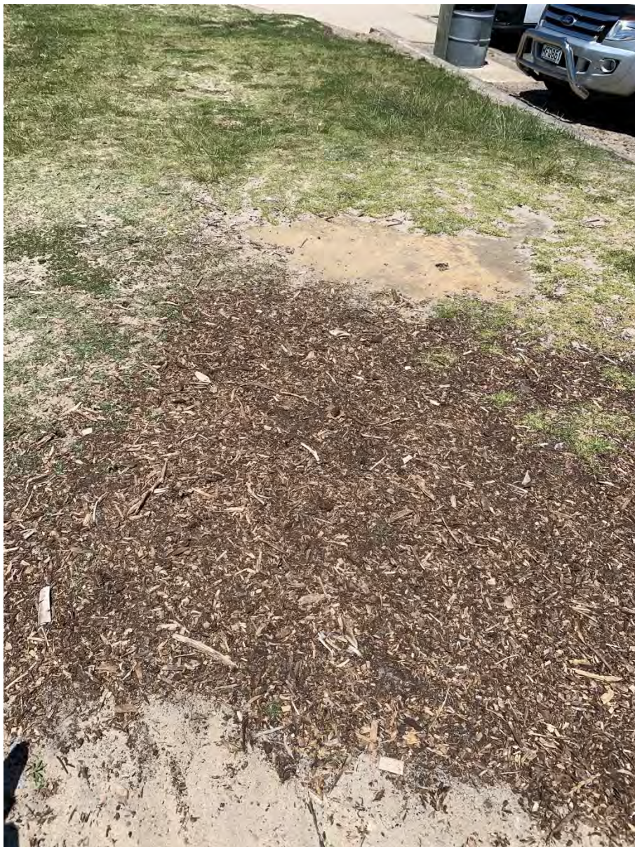
Figure 15: Example of previously consolidated foreshore using clay, rock and bark.
