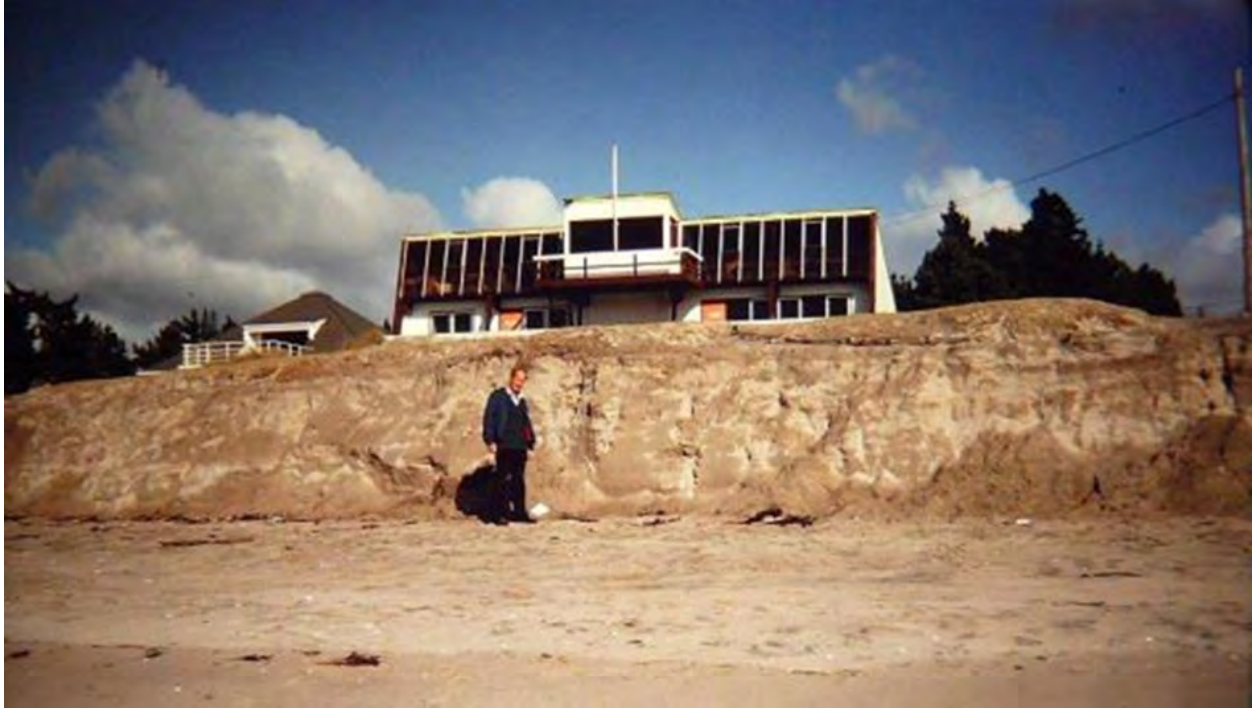
Figure 8: Erosion fronting surf club and Esplanade Dive following the storm of July 1978 (Photo supplied by Ray and Faye Madden)
