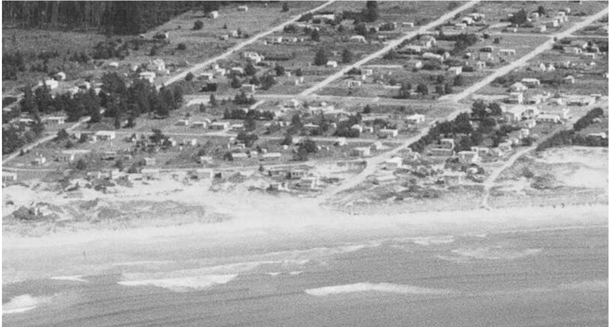
Figure 6: Severe wind erosion damage near the seaward end of Winifred Avenue in 1959 (enlarged from Whites Aviation photo (WA-49858, Alexander Turnbull Library).
