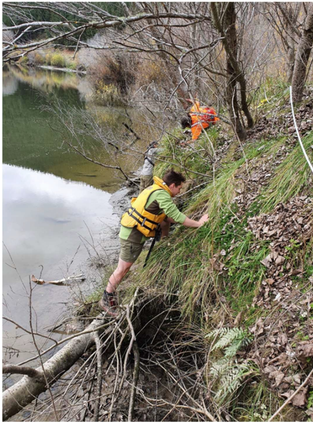
Photo 4. Steep unstable banks under poplar trees.
