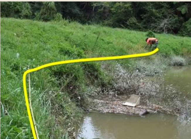
Mateongaonga Stream about 80 m upstream of bridge (site 14)
