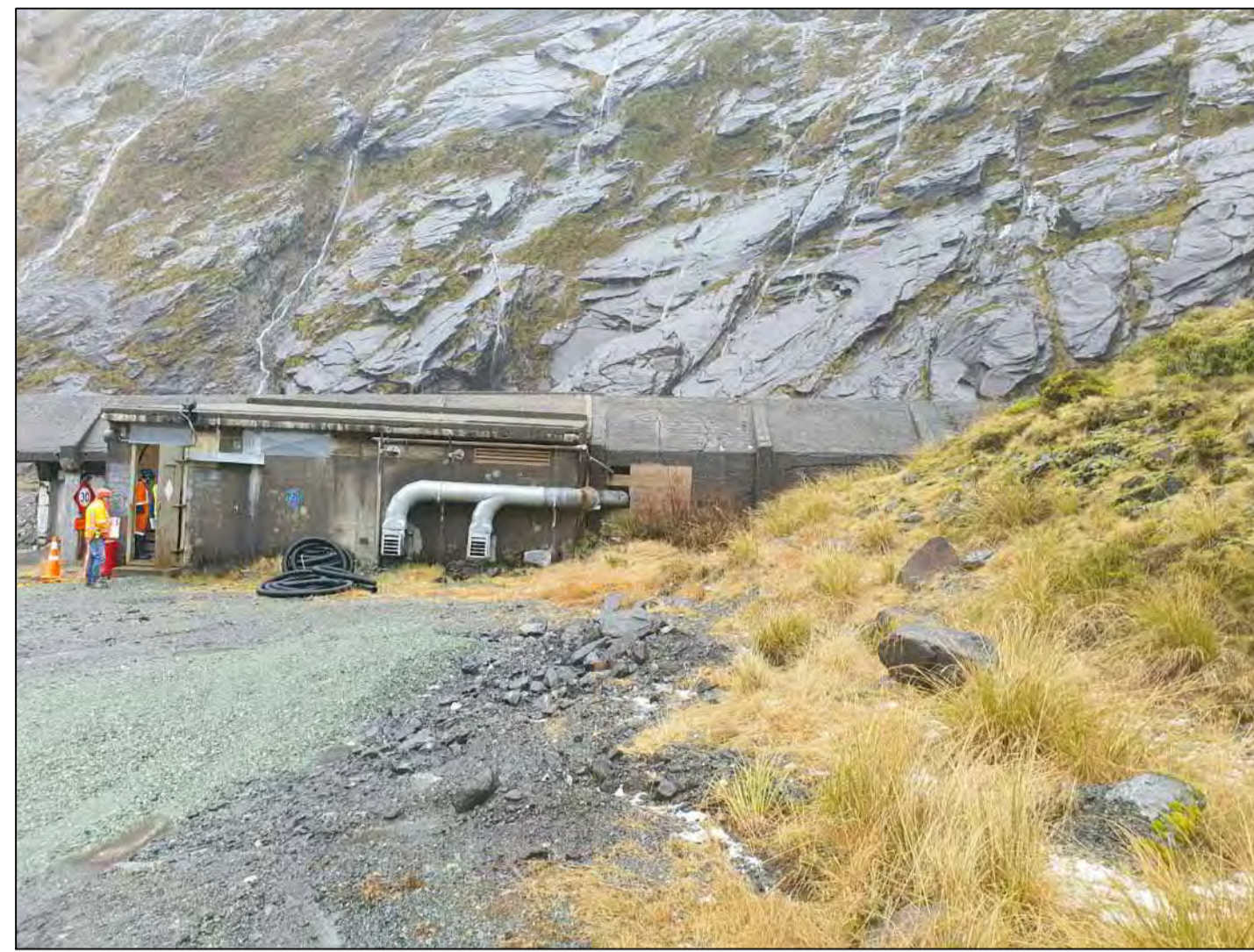
EXISTING AVALANCHE SHELTER AND GENERATOR ROOM
