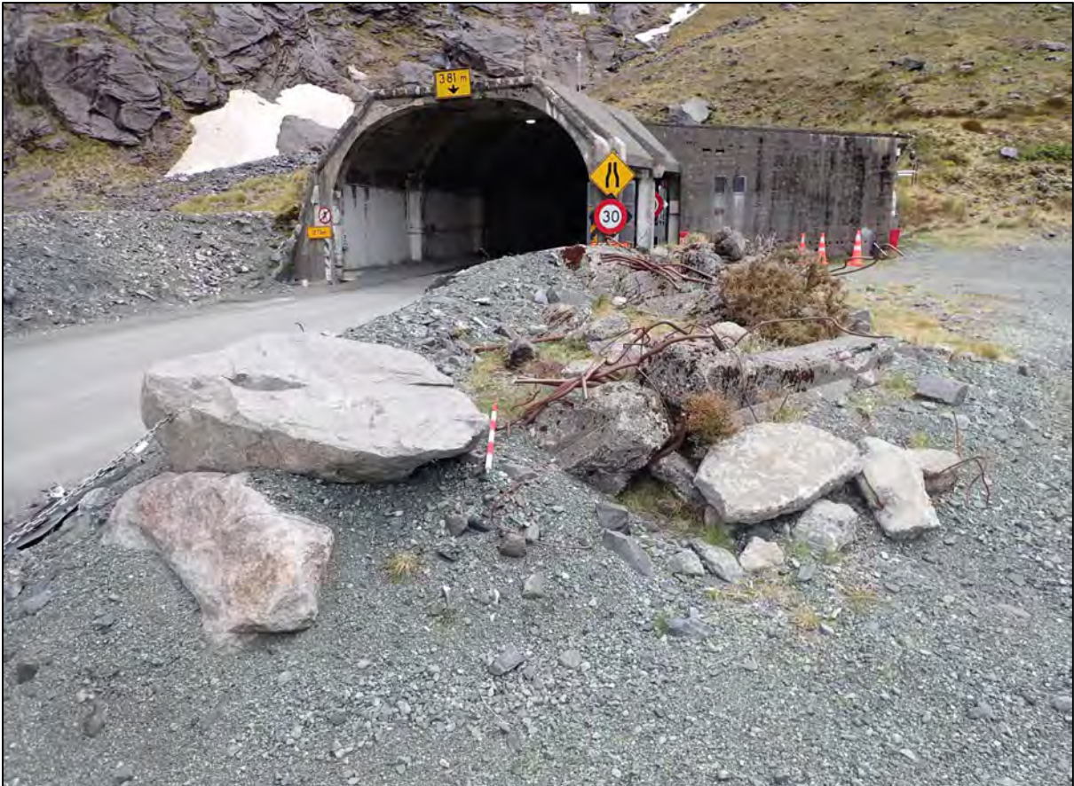
Figure 11. Avalanche debris pile, with the plant room visible behind. 41
