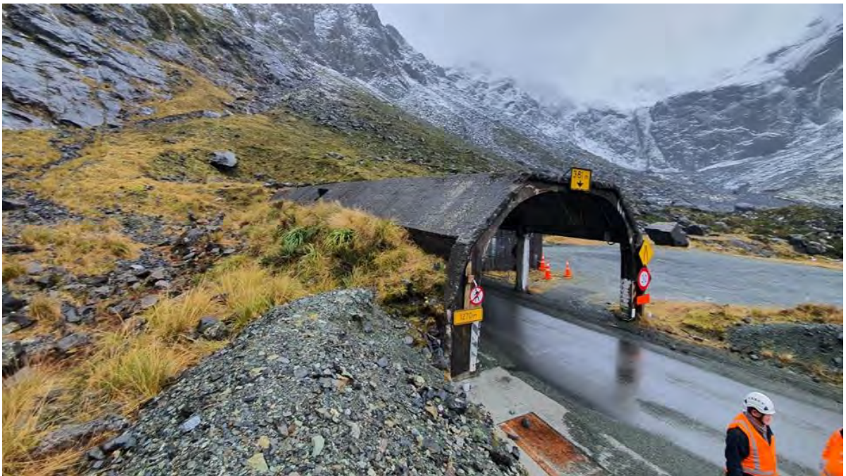
Figure 3-4: View of existing avalanche shelter entrance
