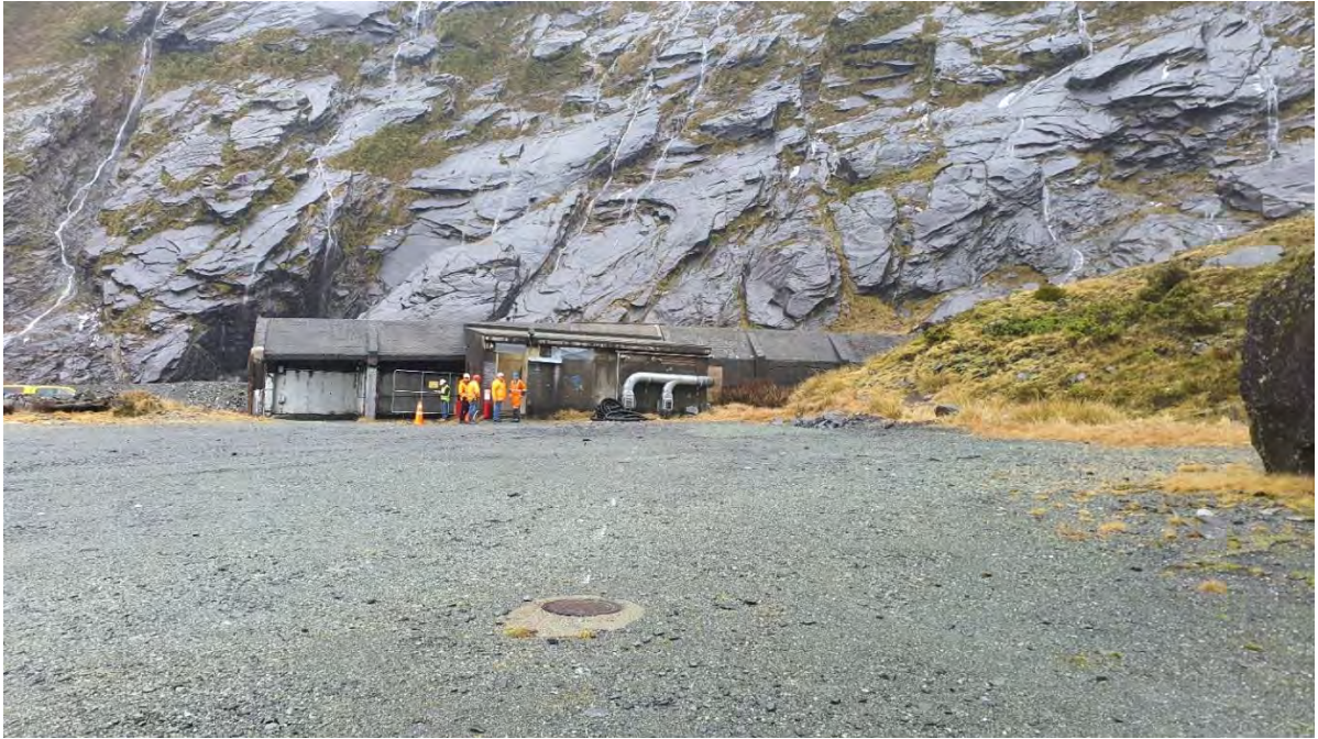
Figure 3-5: Existing avalanche shelter, plant room and talus slope viewed from car park
