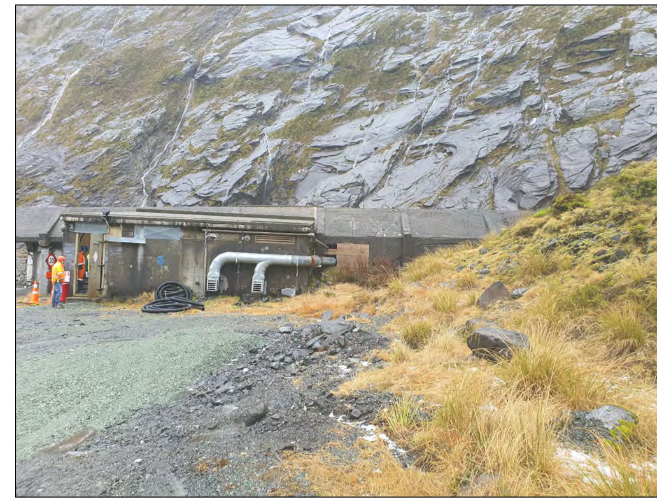
EXISTING AVALANCHE SHELTER AND PLANT ROOM
