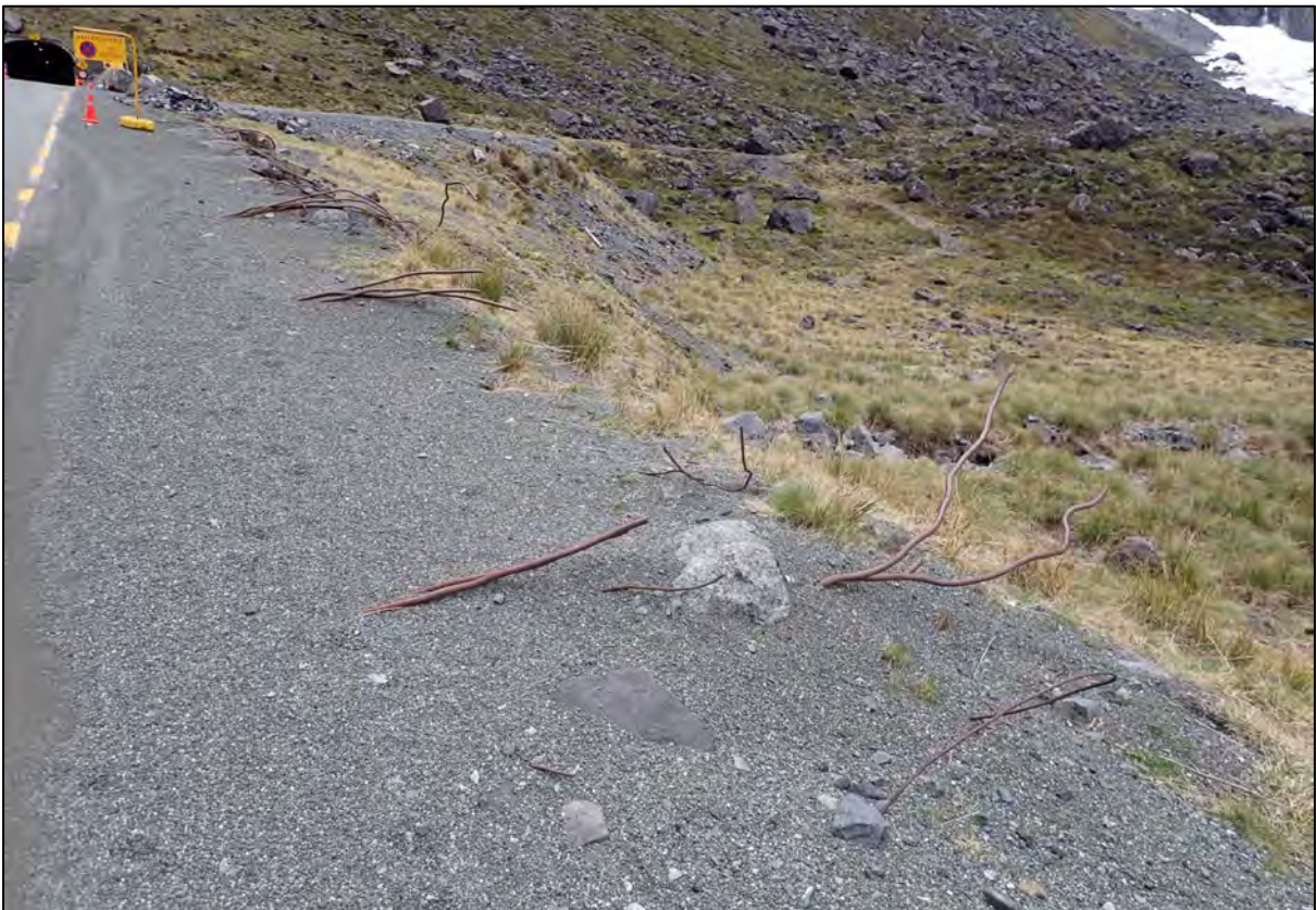
Figure 14. View towards the tunnel, showing some of the avalanche debris along the roadside. 43
