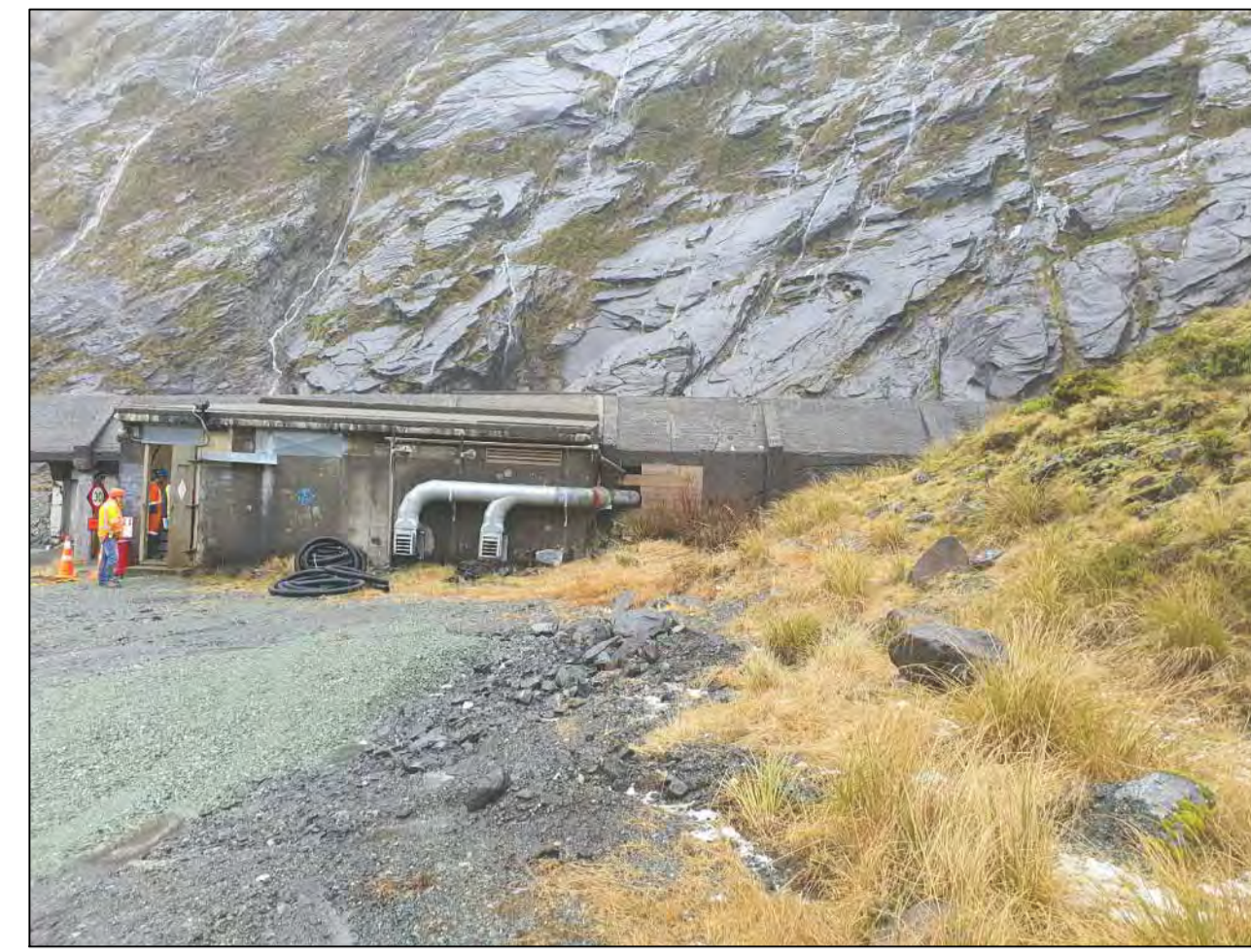
EXISTING AVALANCHE SHELTER AND PLANT ROOM
