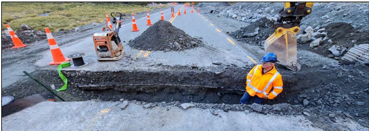
Figure 20. Trenching across the road during the Phase 1 work, looking east.
