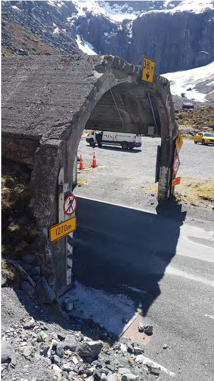
Figure 8-1: Homer Tunnel existing avalanche shelter road entrance
