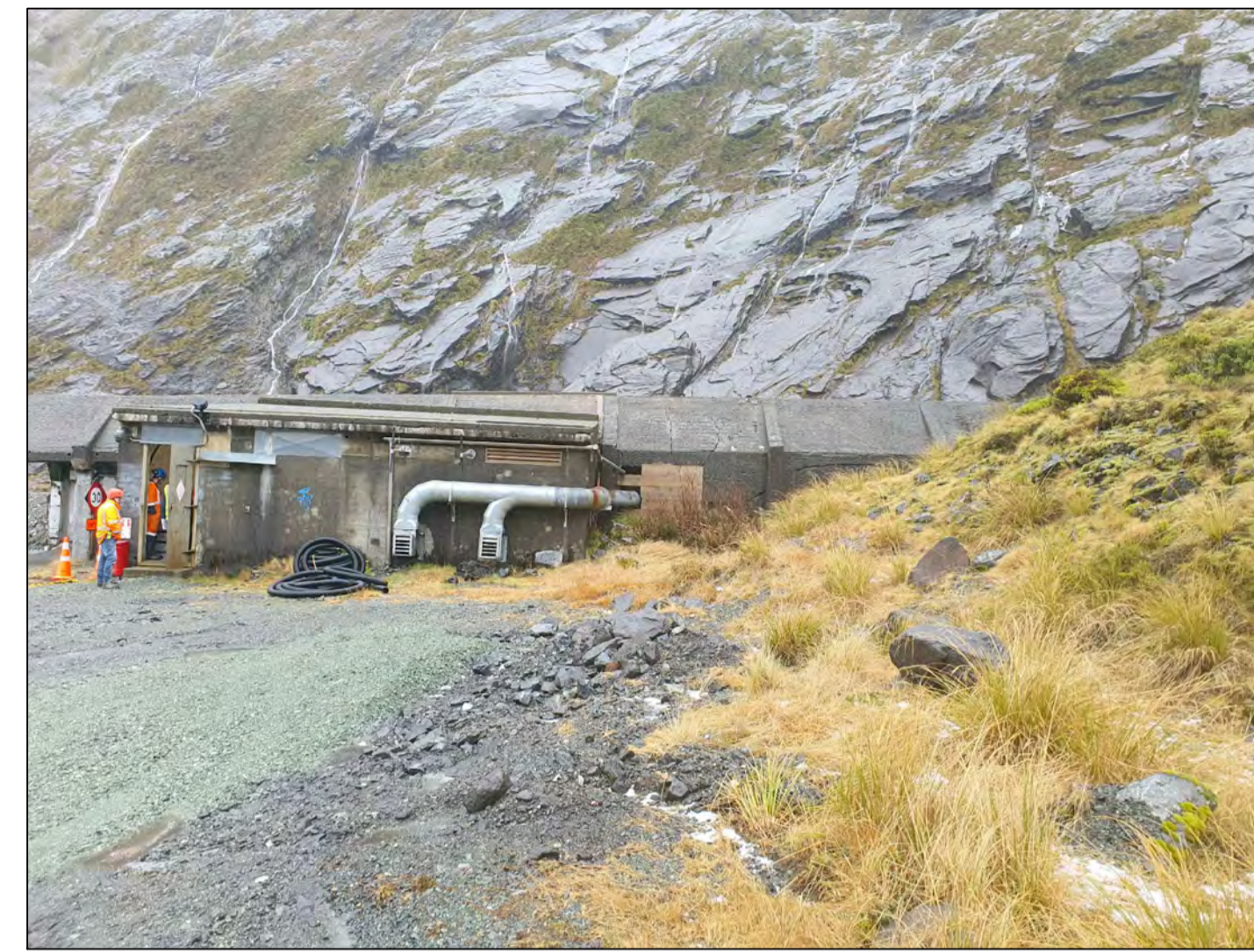
EXISTING AVALANCHE SHELTER AND GENERATOR ROOM
