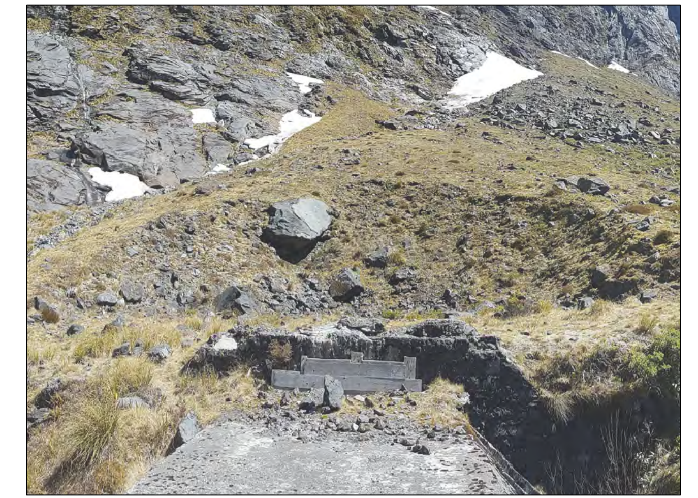
EXISTING PORTAL STONE HEADWALL
