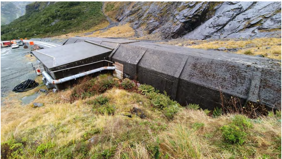
Figure 3-6: Existing avalanche shelter and plant room viewed from talus slope above
