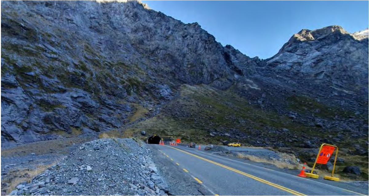
Figure 3-3: Approaching the eastern portal and the existing avalanche shelter, with the dark coloured concrete, existing plant room immediately to the right of the tunnel entrance. There are earth bunds either side of the carriageway. On the left side, the bund provides rockfall protection and the bund on the right side prevents access to the now-closed car park
