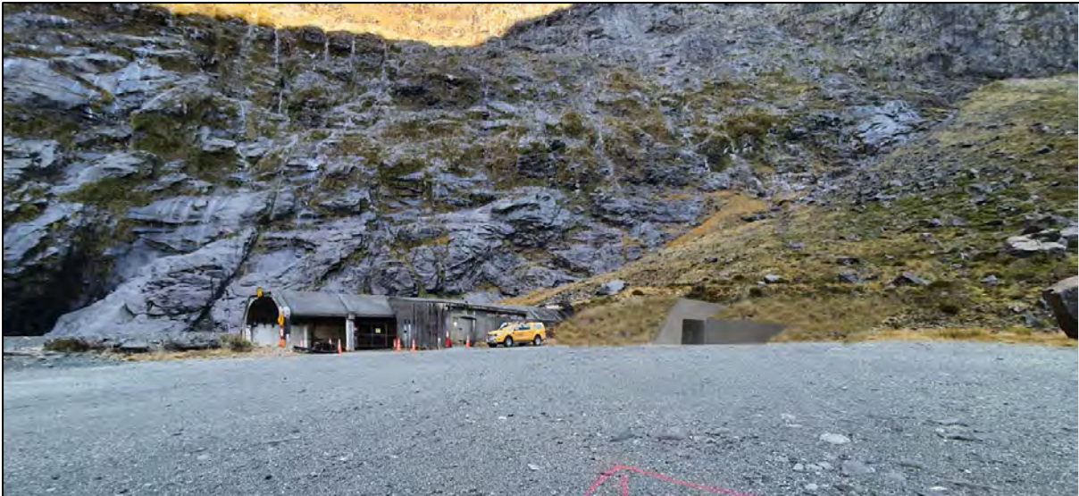
Figure 27. Equipment Building site with render of completed structure.
