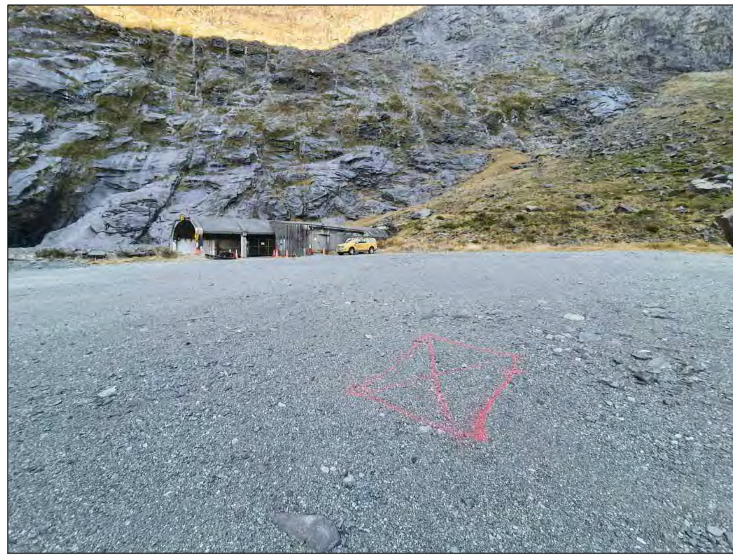
EASTERN TUNNEL PARKING AREA
