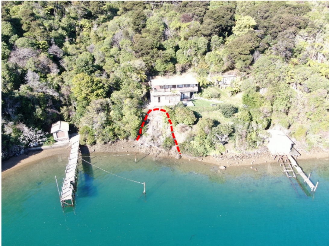
Figure 2: Drone image of the property and landslide
