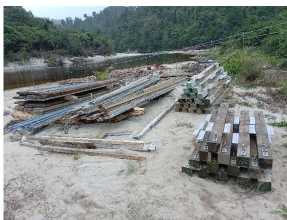
This was a big job. The bridge had over 2000 fixtures, main cables which were 148m long and weighed 360kg each plus a whole lot of wood. The combined weight of material is approximately 12 tonnes (excluding the towers and bridge anchors). All of this was entangled with debris in the river after the storm. Wherever possible, materials will be reused in the new bridge, but regardless, every little piece must be taken out to ensure no waste pollutes the area or endangers wildlife.
