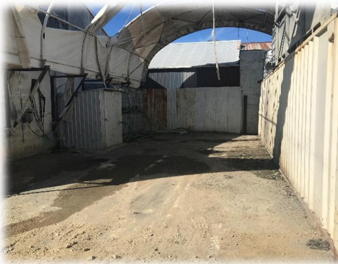
PHOTO 3.15 (f) temp wash bay
