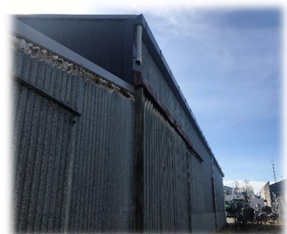
PHOTO 3.10 (e) Southwest end of the building
