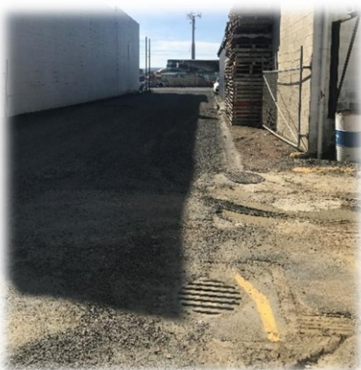
PHOTO 3.14 (f) drive way – catch pit MH-2
