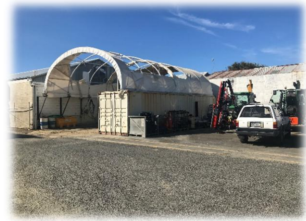
PHOTO 3.13 (f) Southernview temp wash Note: washbay to be decommissioned
