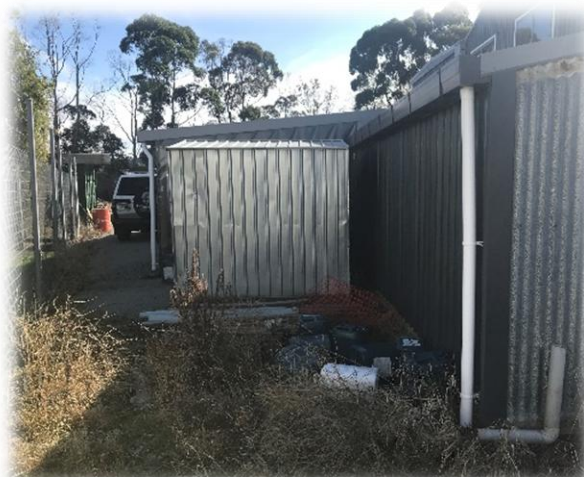
PHOTO 3.9 (e) Southwest end of the building
