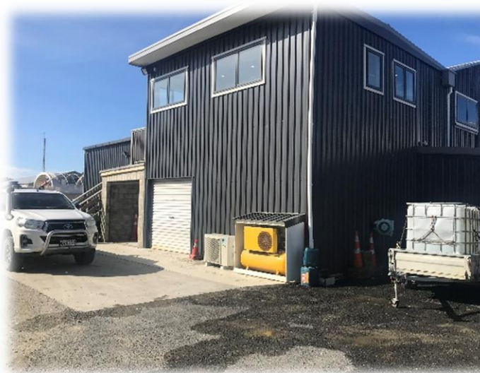
PHOTO 3.6 (b) NW - rear building
