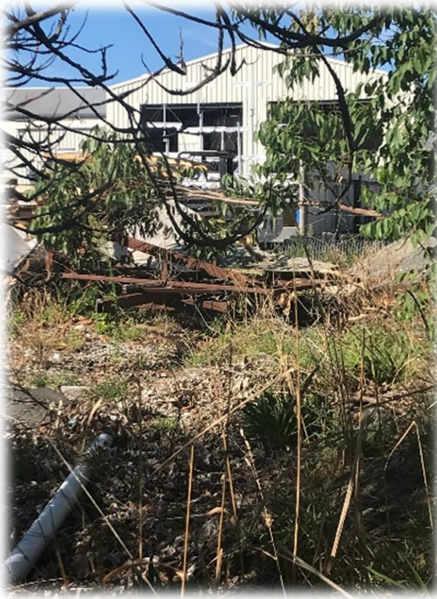
PHOTO 3.20 (i) View from river stormwater outlet
