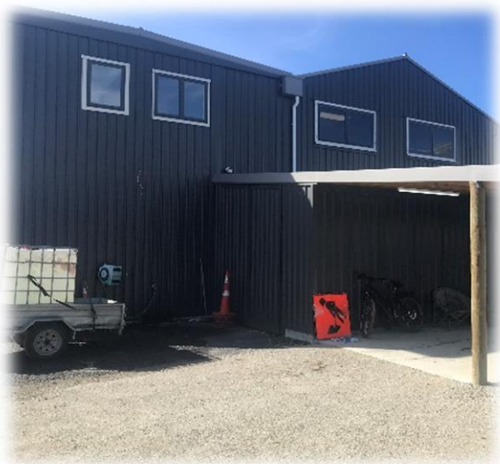
PHOTO 3.5 (b) westerly - rear building
