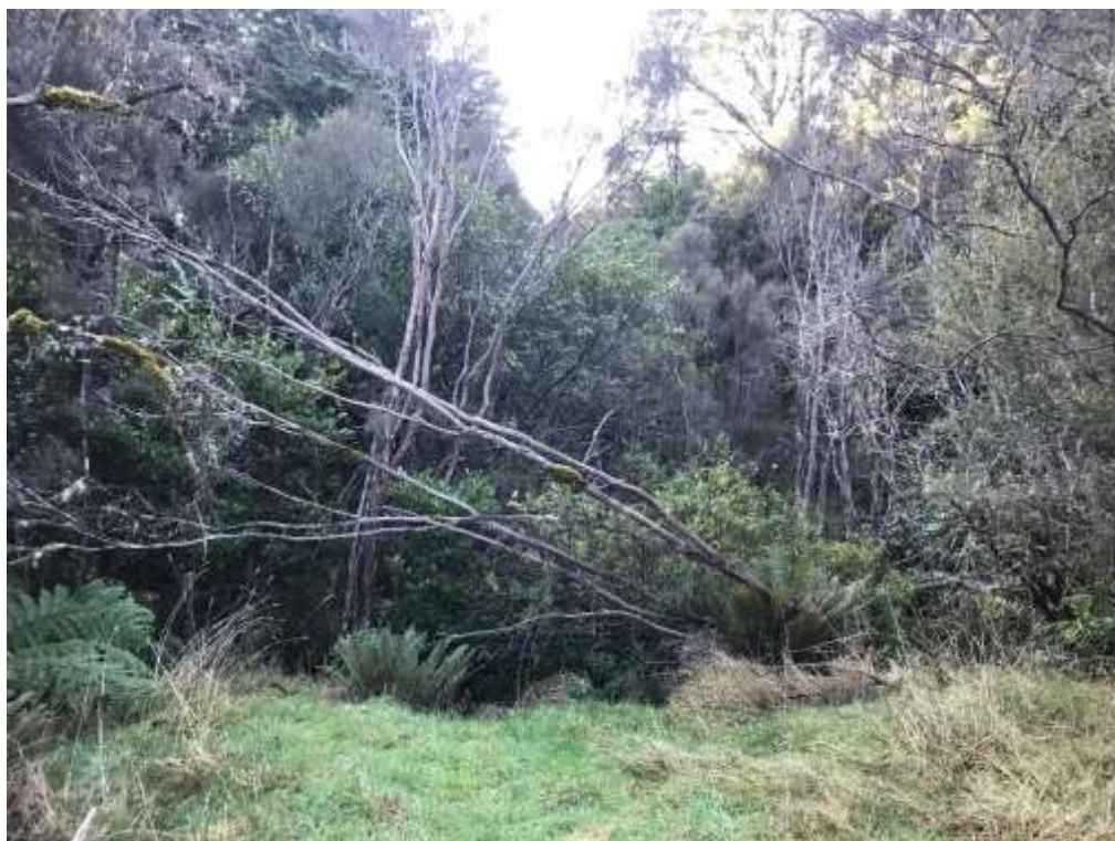
Plate 25: Orautoha Stream in Section 2 of the proposed trail where a new bridge (c.14 metre span) will be required (Section 2.2.B). Concrete struts from an old disused bridge are present here. 23 June 2022.
