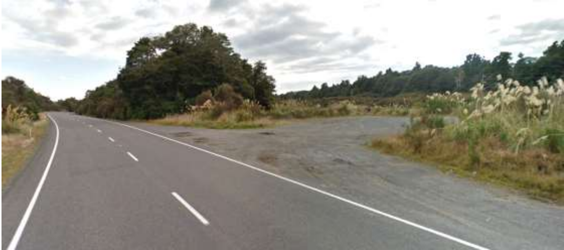
Plate 17: View north from the southern end of Section 5 where State Highway 4 splits from the NIMT railway. The trail will be hidden entirely from view of the State Highway to the north of here.
