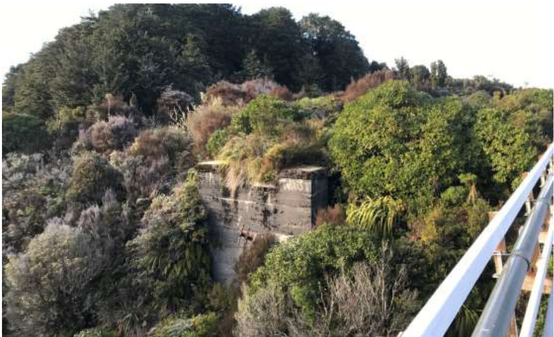
Plate 21: View southwards from the rail bridge. The trail will go around the old bridge abutment and cross under the rail bridge here, before rising back into beech forest on the right side of the rail bridge. Care will be required at this location, to minimise clearance, earthworks, and ensure structures fit into the landscape.
