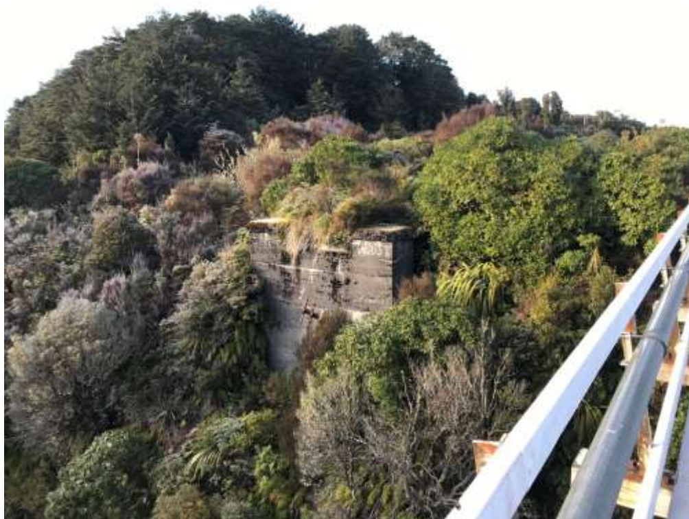
Plate 18: View of old bridge abutments on the southern side of Manganui-o-te-Ao River, with orihou shrubland in the foreground (Section 7.1.W of the proposed trail). NIMT rail bridge is visible in the right-foreground. 23 June 2022.
