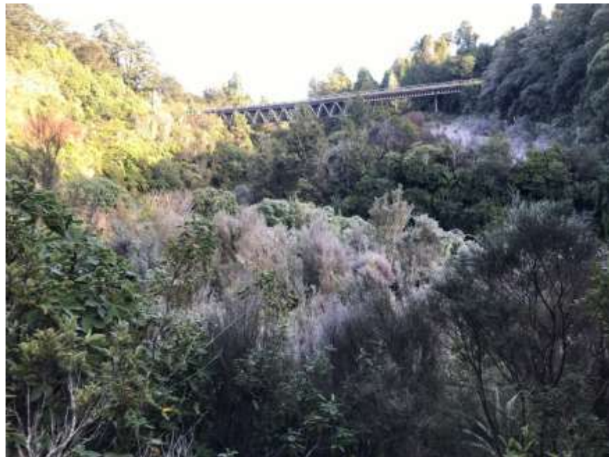
Plate 17: View from the southern side of Manganui-o-te-Ao River, with mānuka scrub in the foreground (Section 7.4.B of the proposed trail) and exotic grassland on the northern side of the river (Section 7.5). State Highway 4 bridge is visible in the background. 23 June 2022.
