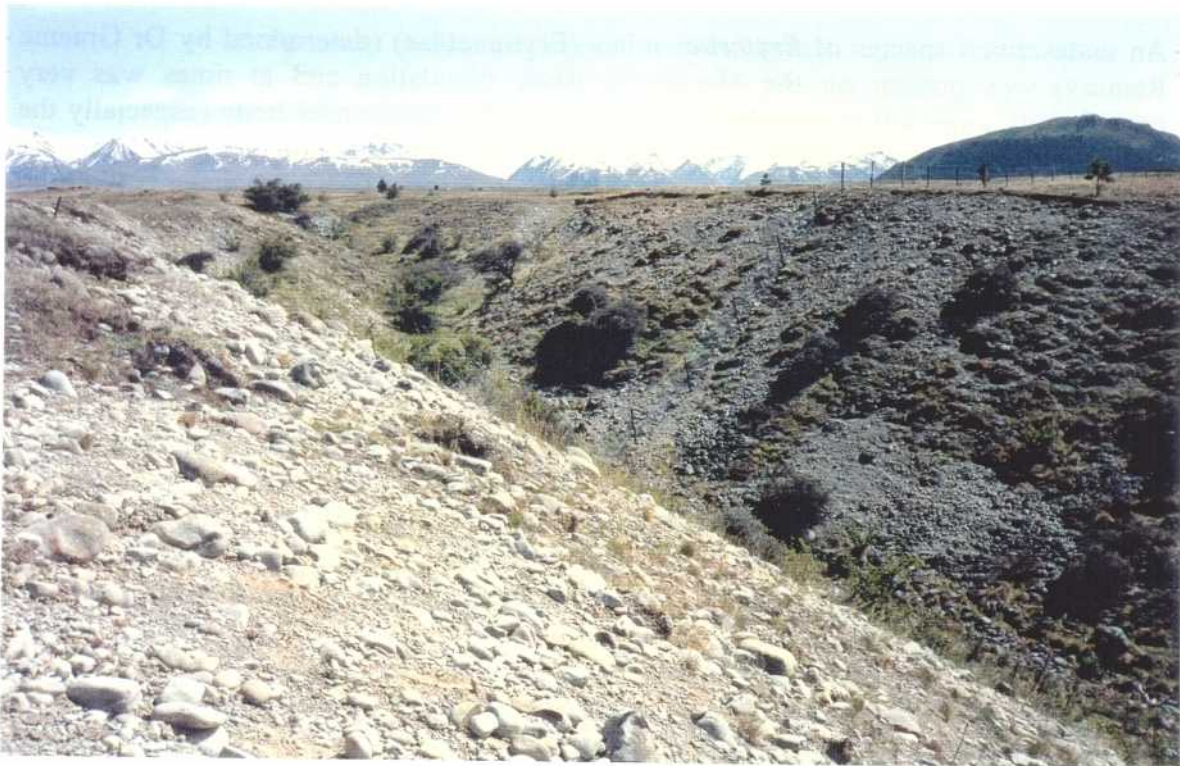
Figure 9 Tekapo Canal, high terrace lateral gully showing degrading embankments of fluvioglacial deposits.
