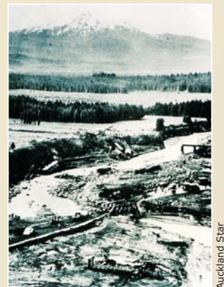
Tangiwai rail disaster caused by bridge collapse during dam-break lahar in 1953.
