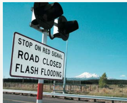
Automatic lights are installed on State Highways 1 and 49.
