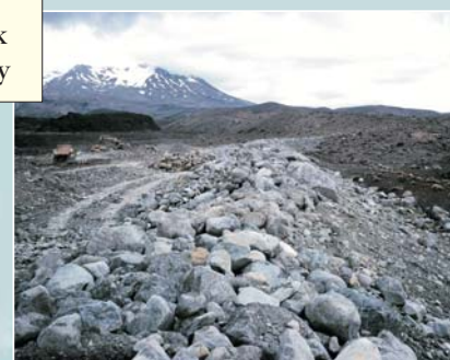
The 300-m-long bund under construction
