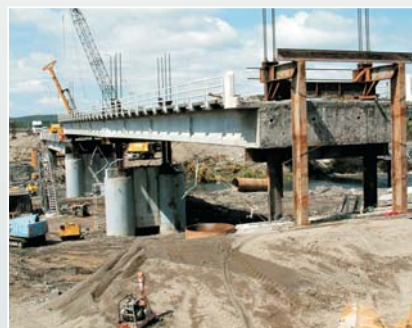
State Highway 49 bridge being raised and strengthened.
