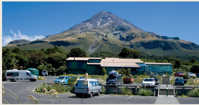
Taranaki/Egmont National Park Visitor Centre. Photo: Tim Weston
