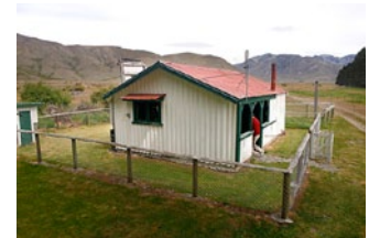
Red Gate Hut.
