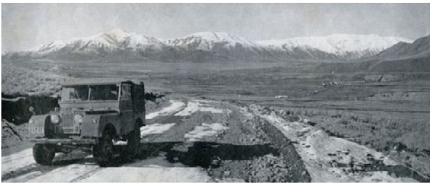
The 'new' road above Sedgemere linking North Canterbury and Nelson via the upper Clarence Valley and Island Saddle, built to serve the construction and maintenance of the 1958 line. An electricity workers' camp with a line of huts can just be seen in the middle distance at right.
