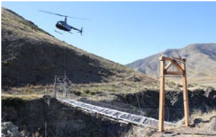
Moving materials to the other side.
