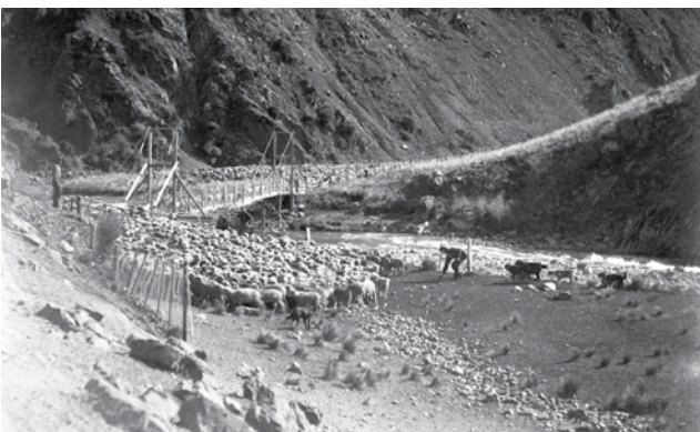
1. Saxton River stock bridge.
