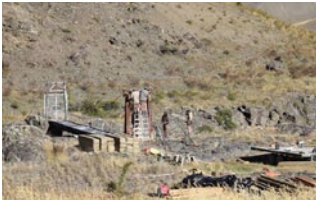
Starting to renew the first tower.
