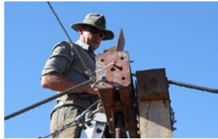
Assembling a new tower.
