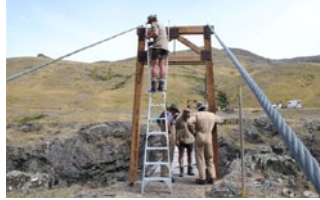
Putting finishing touches to the second new tower.
