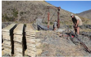
Using a turfer winch to position parts.
