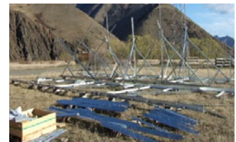
Assembling a new transmission structure.
