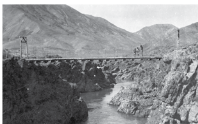
4b. Second bridge on the same site at the mouth of the Acheron River – Engineering Students' Stock Bridge.
