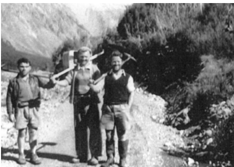
A pylon foundation digging gang possibly in the Upper Wairau 1957.
