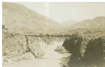
4a. 1890s stock bridge at the mouth of the Acheron River.
