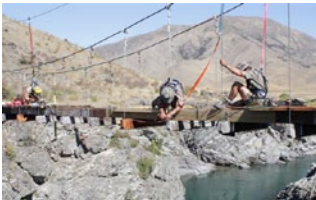
Strapped into safety harnesses while working on the deck.
