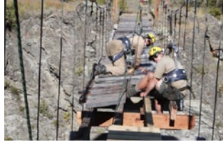
Replacing decking.
