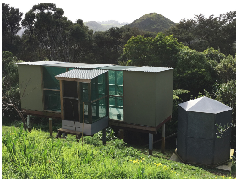
Figure 5. Flight aviary showing sheltered ends, shade cloth walls and a secure entry-way. Note metal predator control wrapping on piles. Photo: Karen Saunders.
