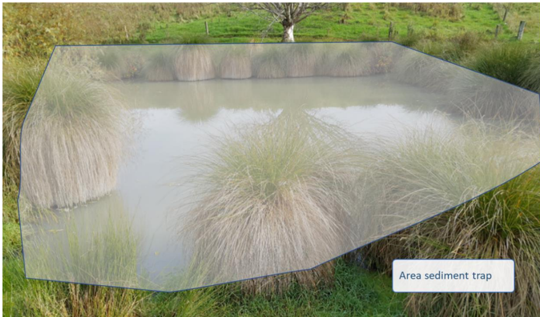
Figure 10. The area of an established sediment trap. Image source: www.es.govt.nz .
