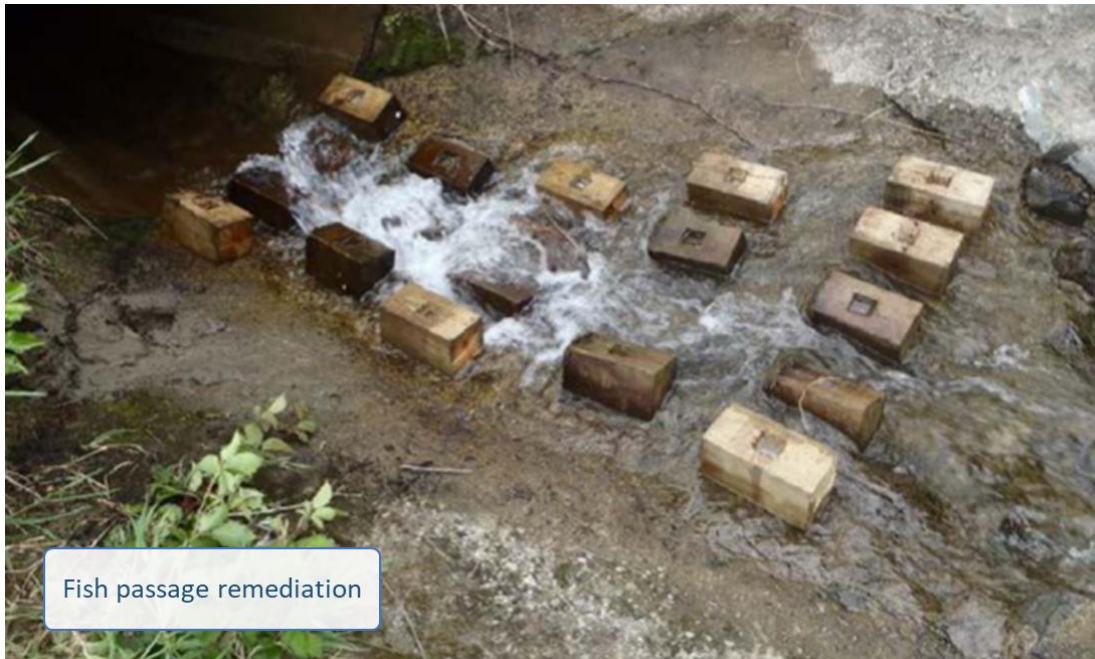
Figure 12. One type of fish passage remediation activity, with blocks creating variable flow areas, and resting spots for migrating fish. Image source: Franklin et al. (2018).
