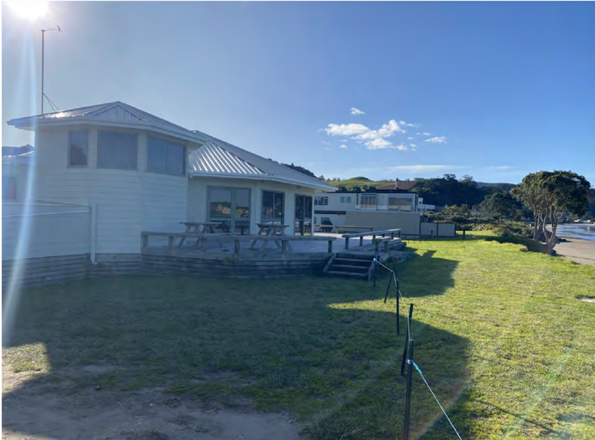
Figure 5 - Clubroom building at existing site immediately prior to the 2023 cyclone events.
