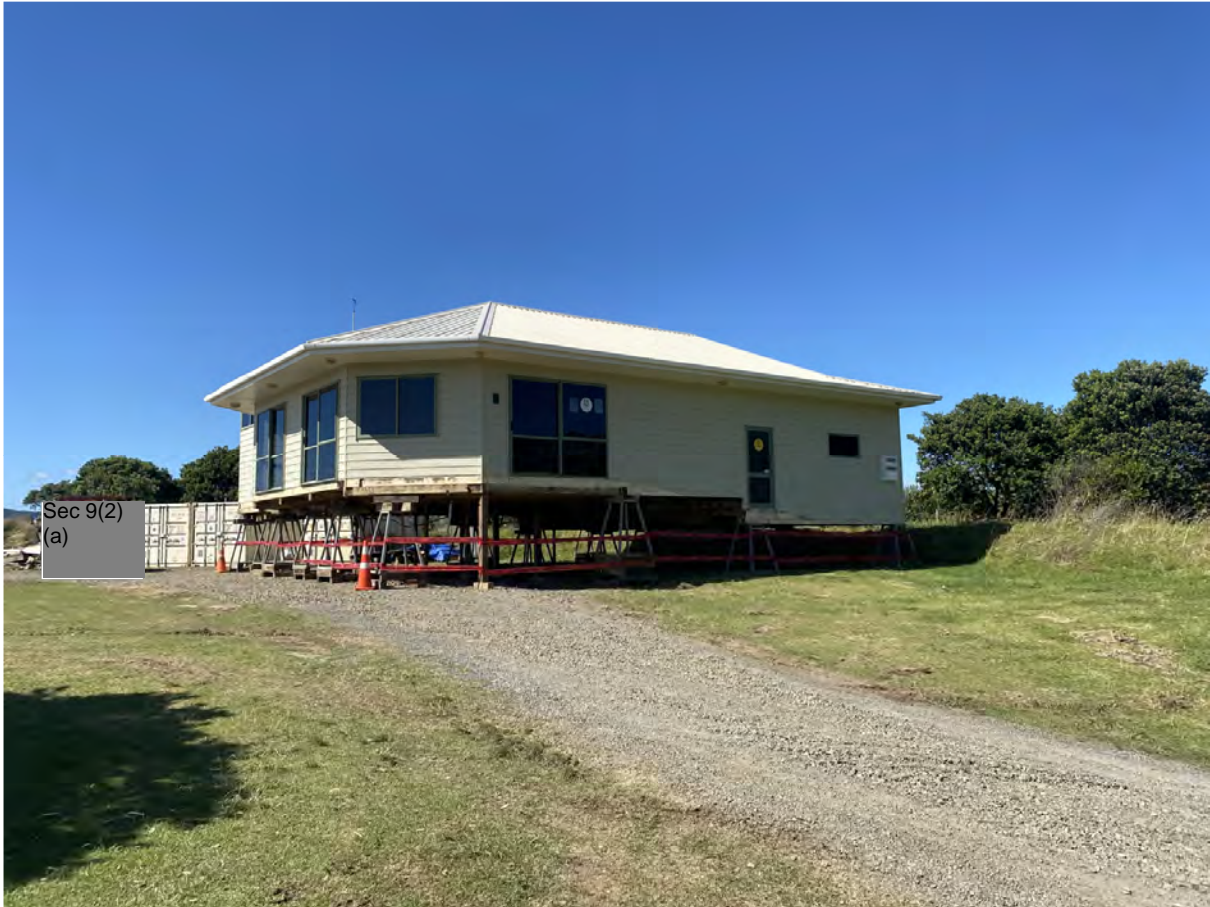
Figure 8 - Clubroom building currently on temporary stands at Buffalo Beach.
