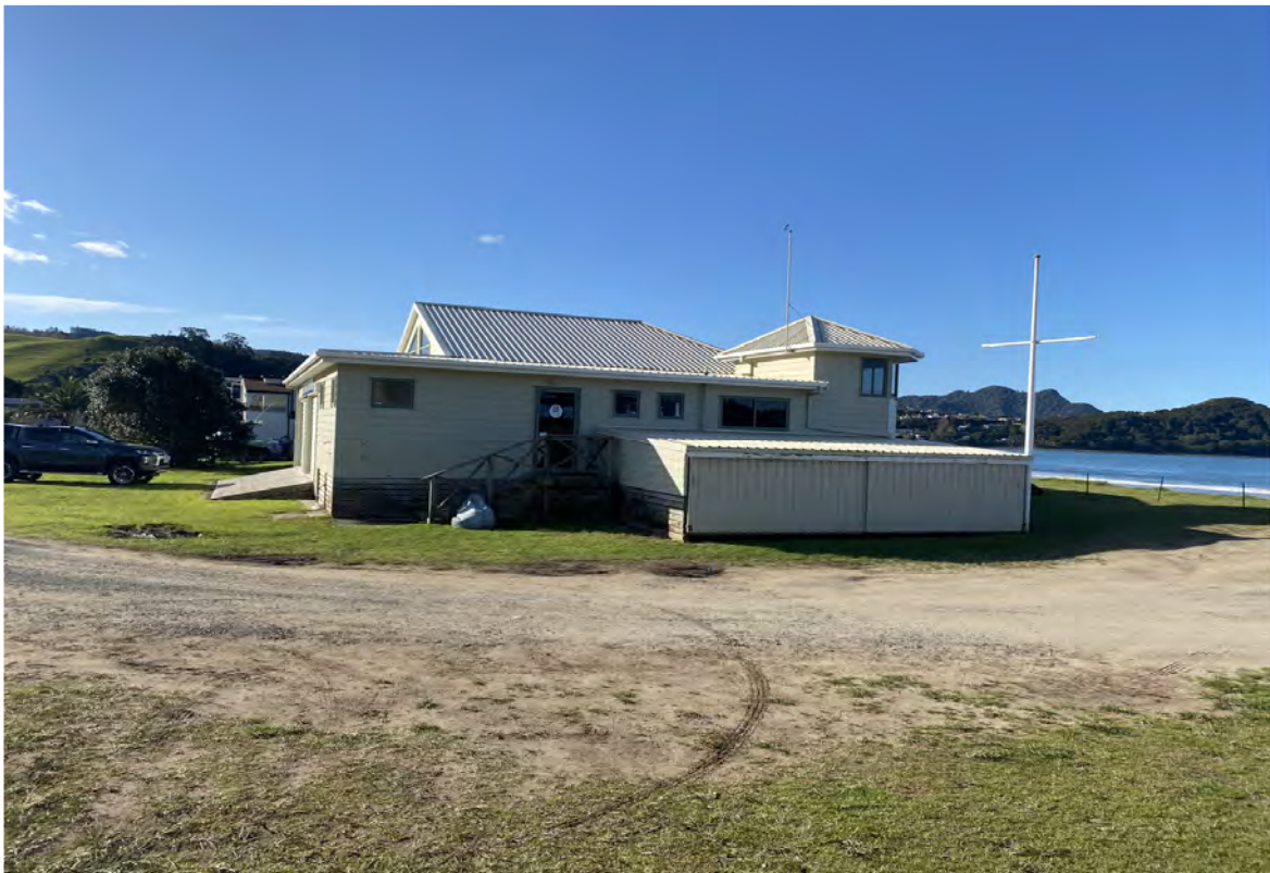
Figure 4 - Clubroom building at existing site prior to the 2023 cyclone events.
