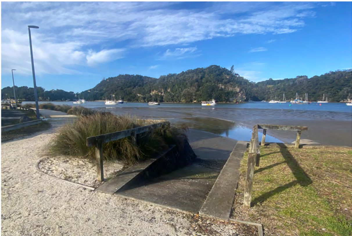
Figure 9 - Public kayak ramp on the northern reclamation.
