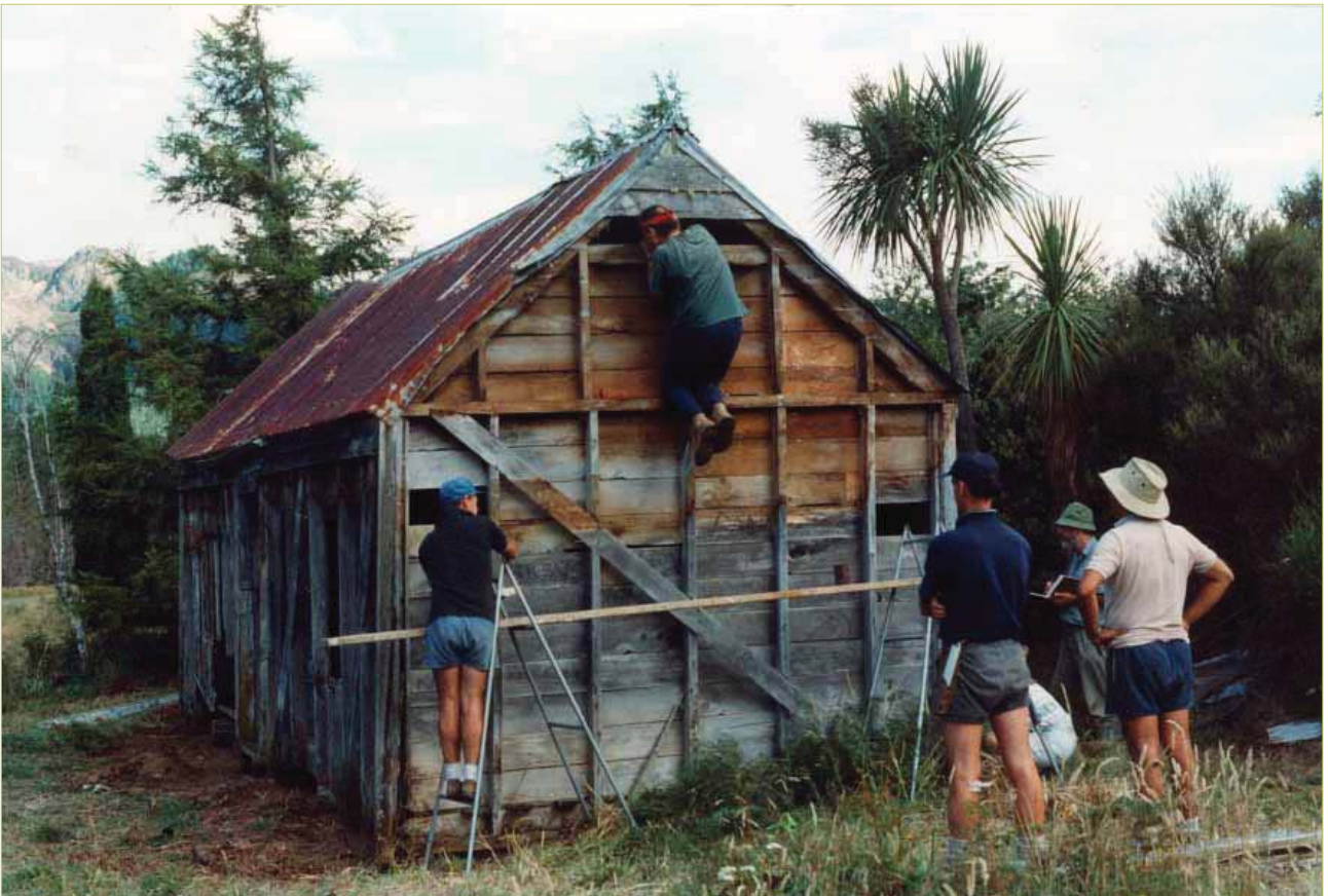
FIGURE 7: BUILDING TECHNOLOGY TEAM AT WORK ON THE WEST WALL
