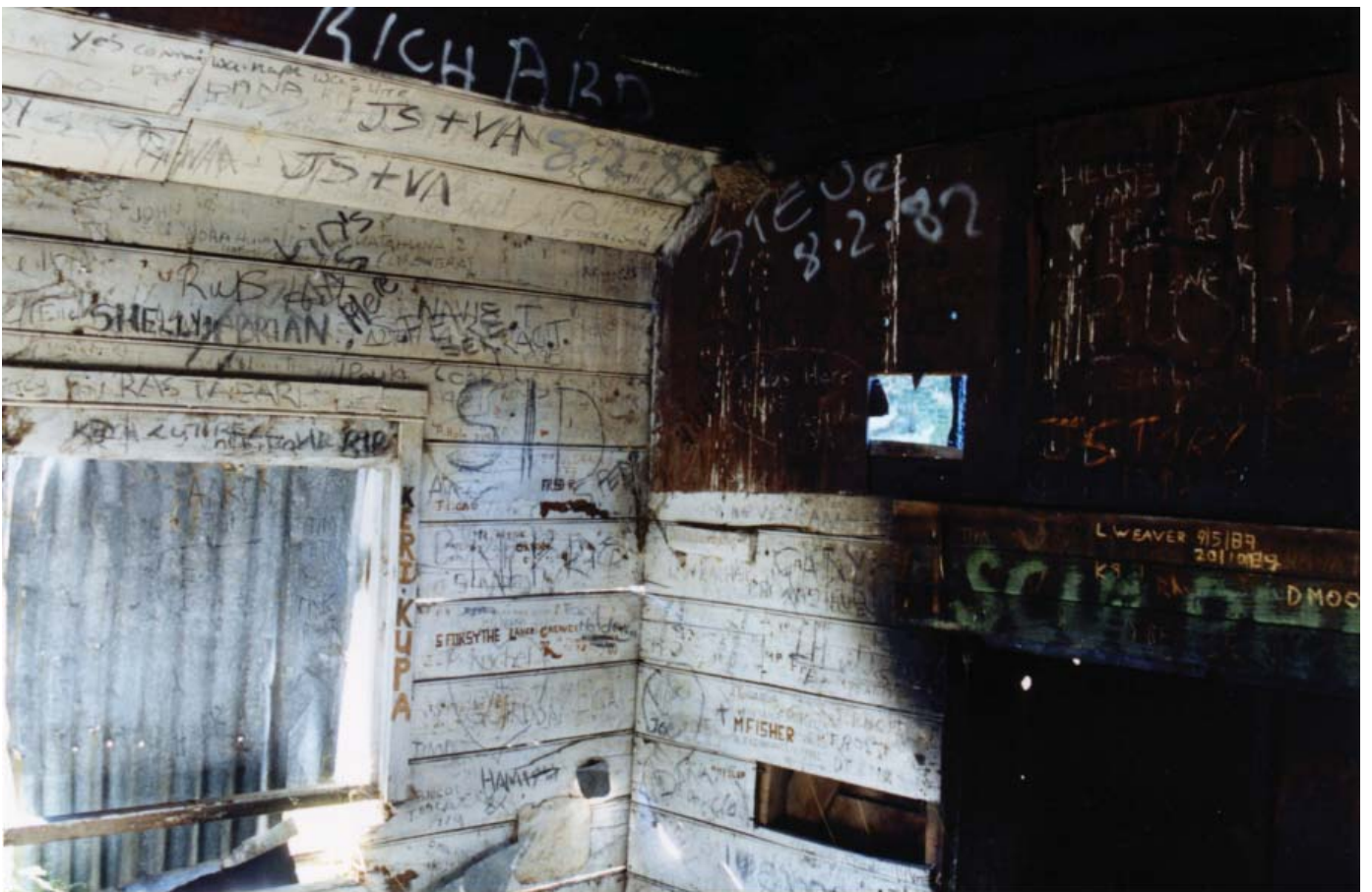
2 Interior, main room. Fireplace on the right.
