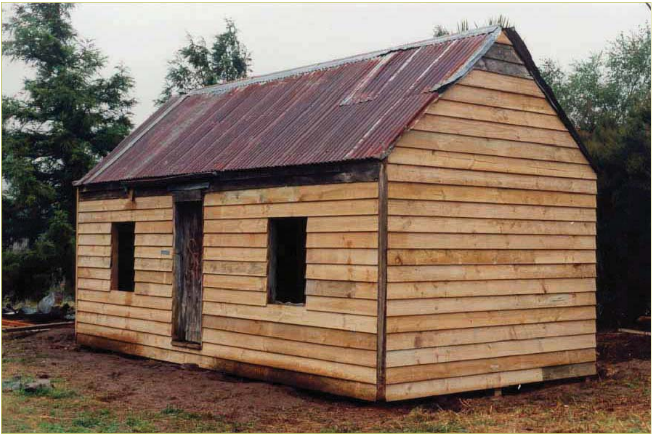
FIGURE 18: PINE CLADDING ON NORTH AND WEST WALLS
