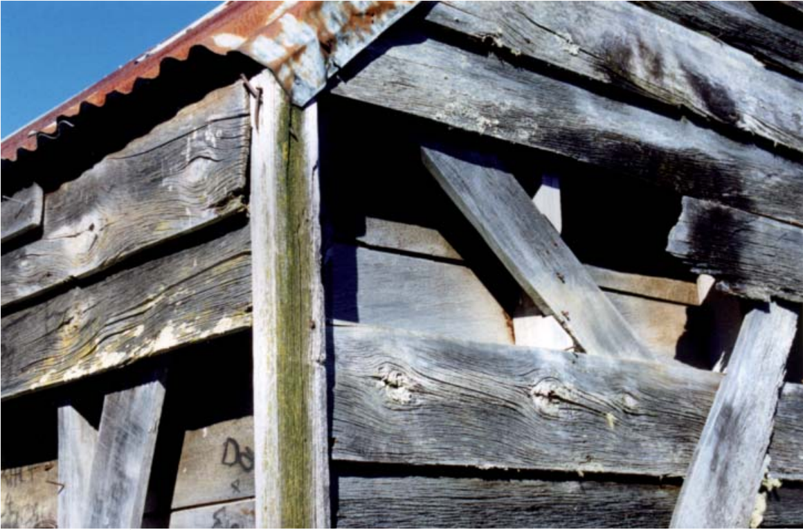
Detail of solid corner stop, north corner.
