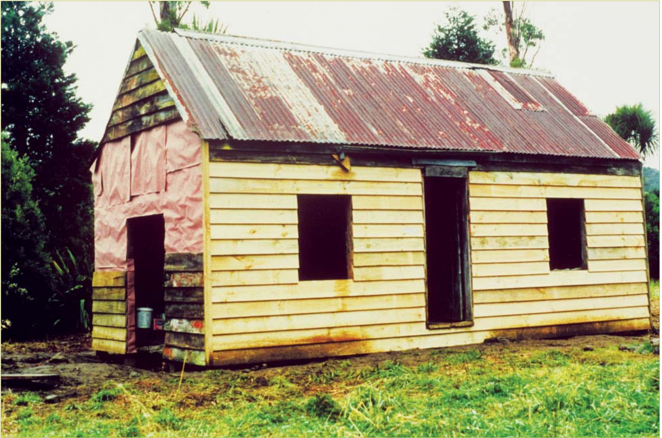
FIGURE 16: PINE CLADDING ON NORTH AND EAST WALLS
