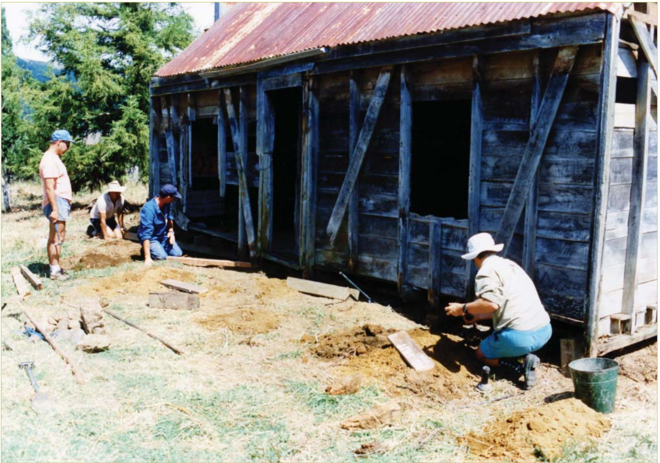
FIGURE 12: REPILING NORTH WALL
