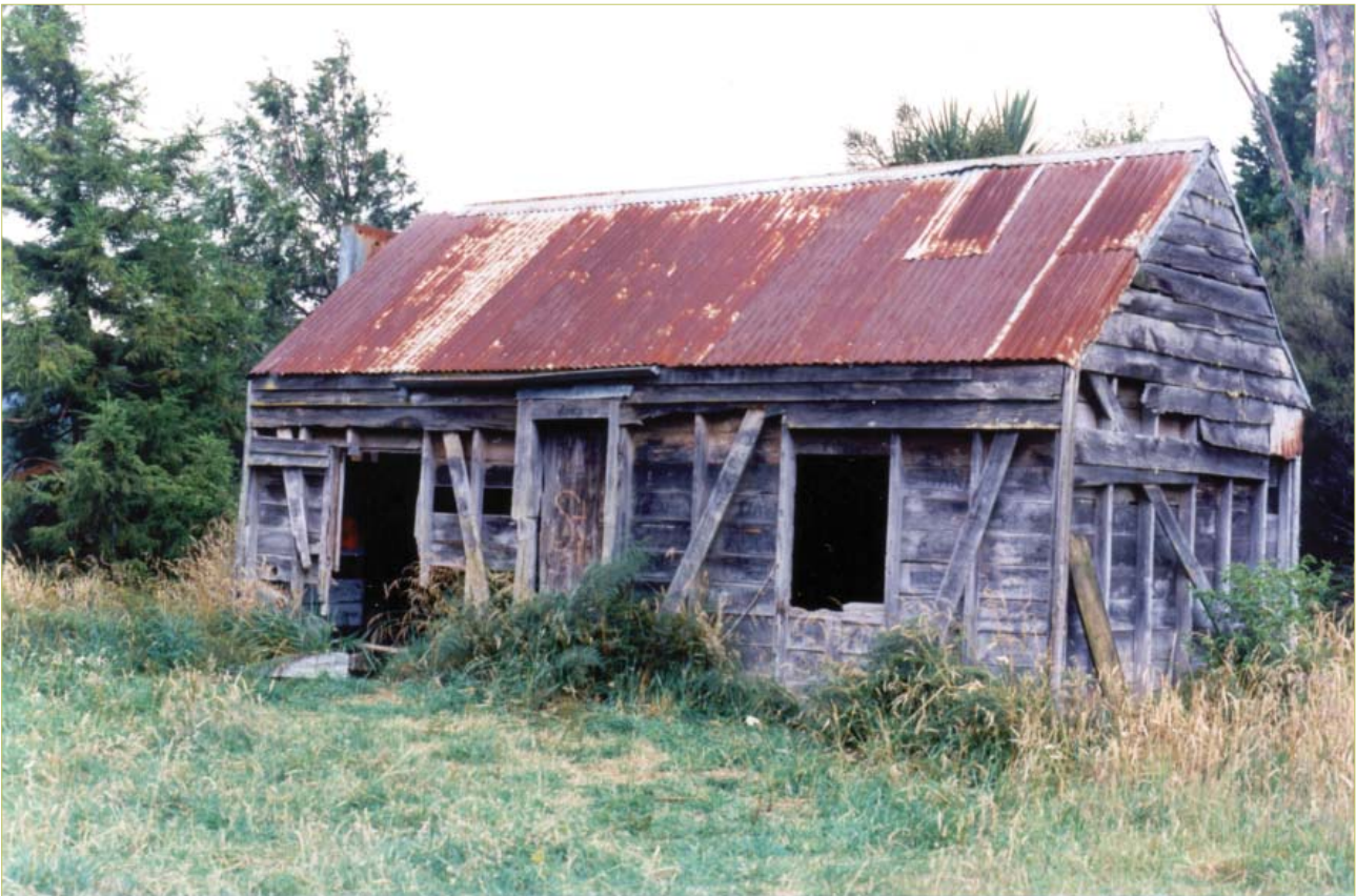
FIGURE 5: ELLIS HUT BEFORE CONSERVATION
