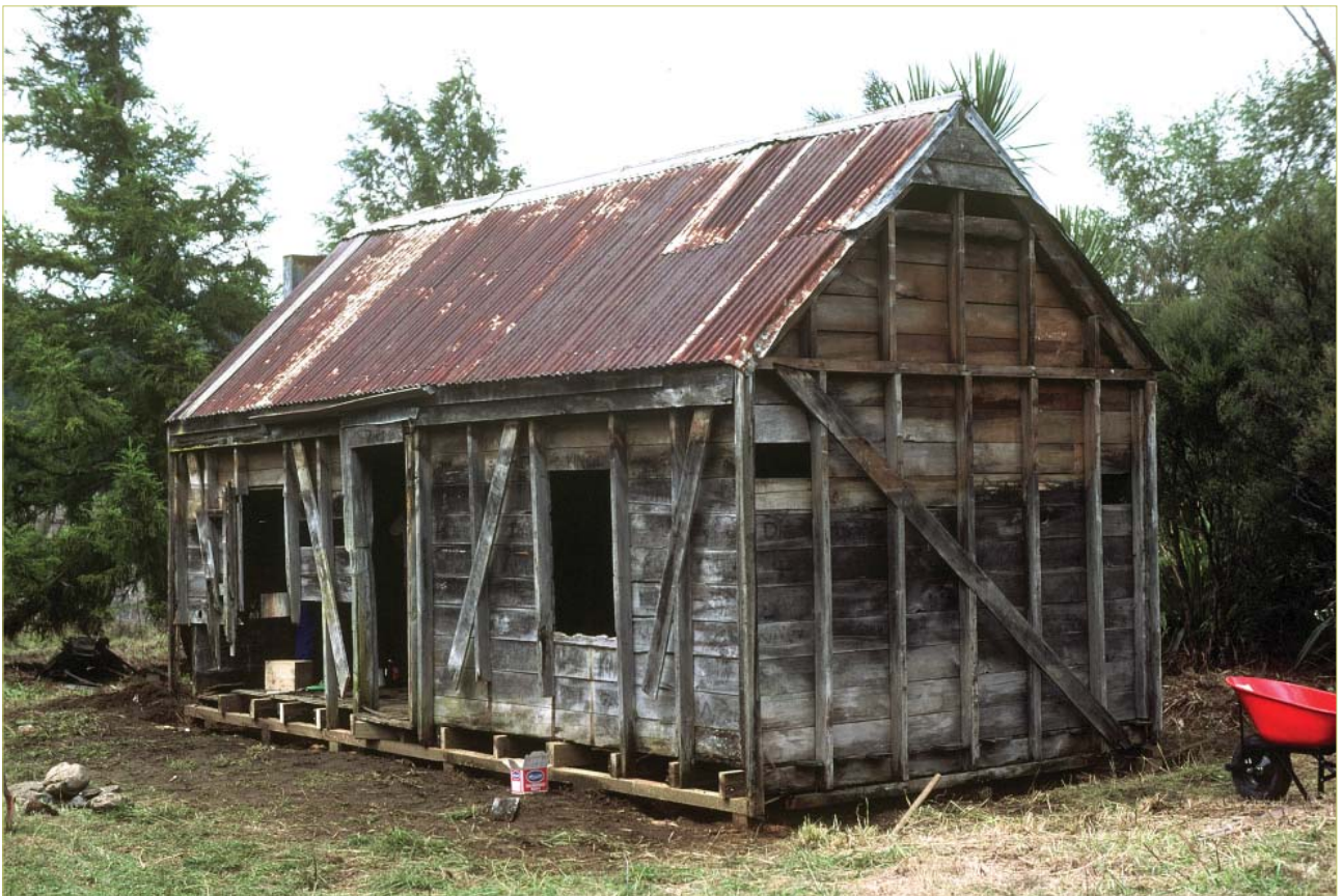
FIGURE 13: REPILING COMPLETED
