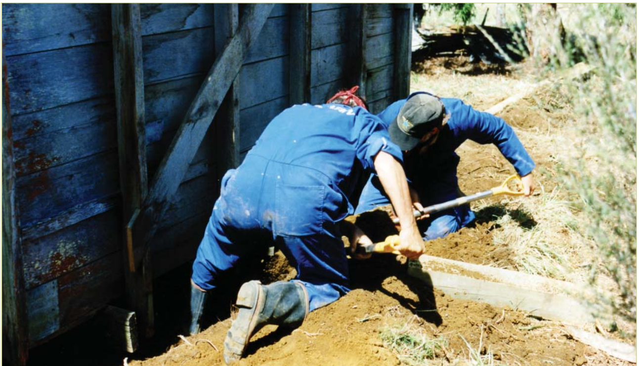
FIGURE 11: HUT BEING LEVELLED
