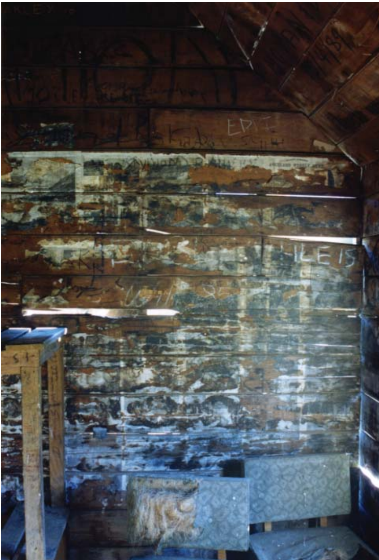
← Detail of boarding in bunk room. 4
