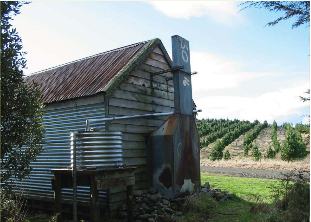
FIGURE 17: NEW WATER TANK AND REPAIRED CLADDING ON EAST AND SOUTH WALLS
