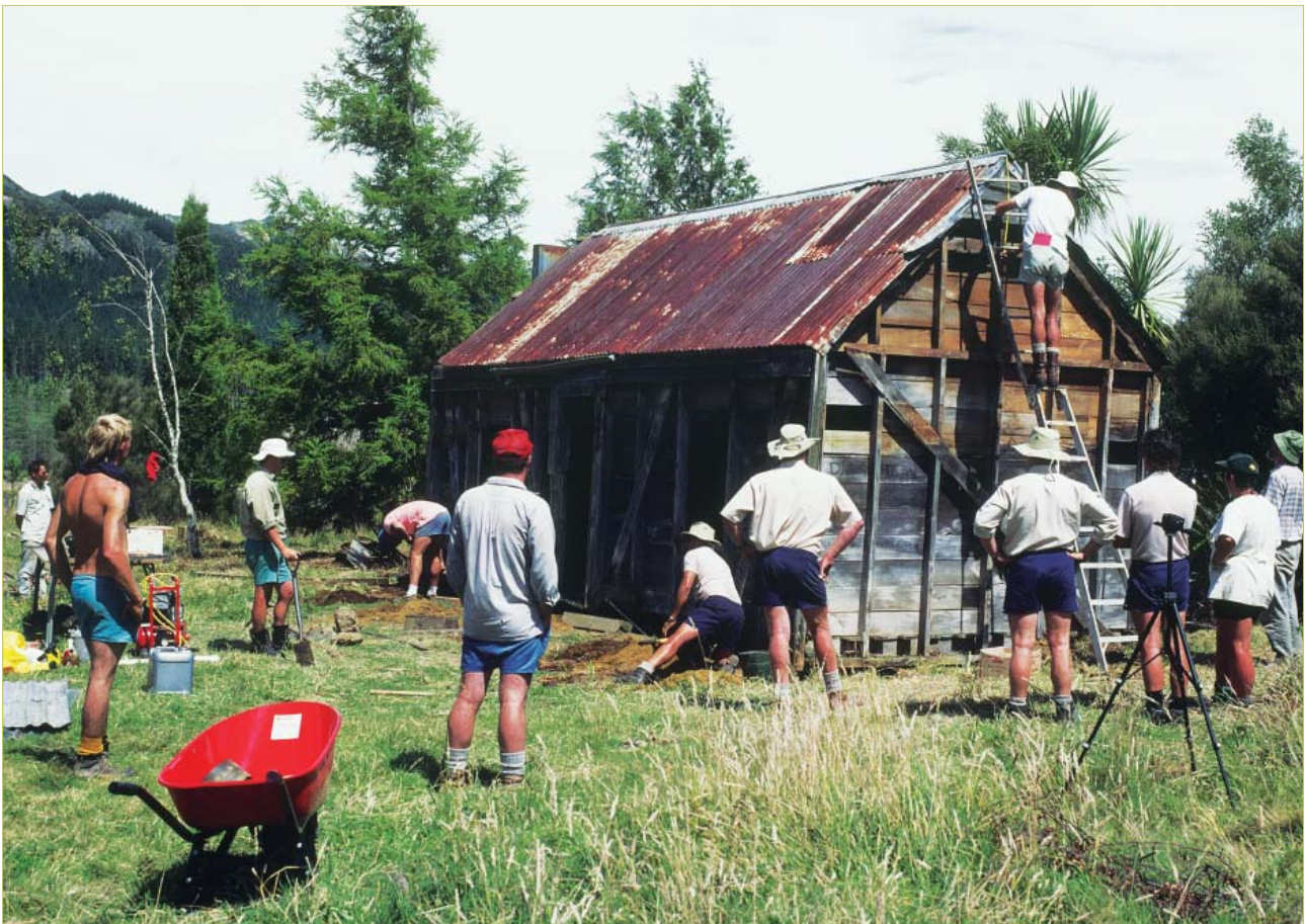
FIGURE 6: WAITING FOR THE TECHNICIAN'S ADVICE
