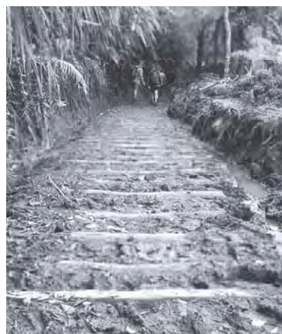
Work in progress on the Waitawheta Track. Photograph: DOC.
