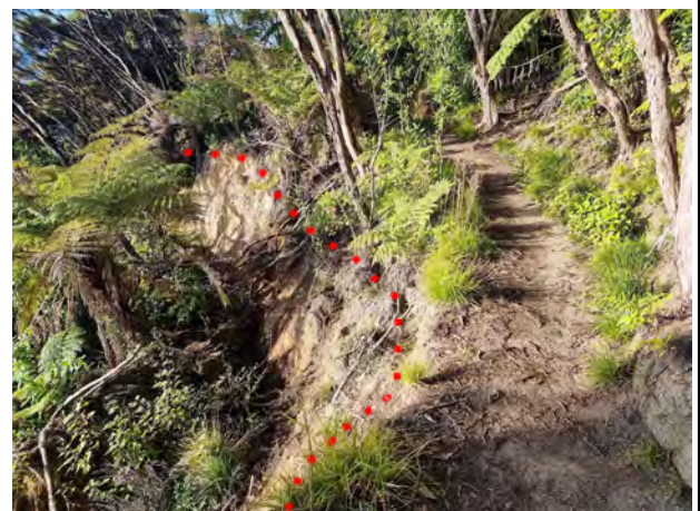
Figure 30. Newly constructed track with the headscarp of the large landslide immediately to the left, showing that the track is highly likely to be damaged in the near future. Headscarp indicated with a red dashed line.
