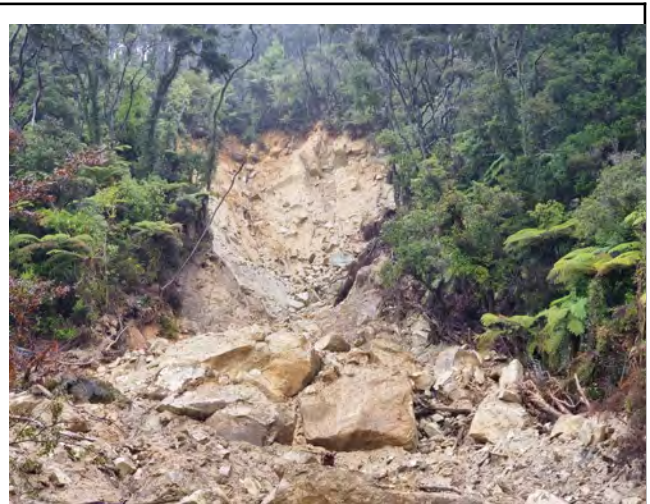
Figure 8. Large scale rockfall at Bark Bay.
