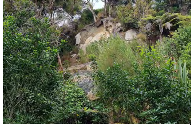
Figure 12. Rockfall at the Anchorage hut and campsite.
