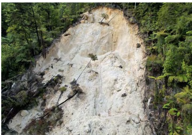
Figure 5. Large translational slide with complete soil displacement at the Torrent River swing bridge (Cleopatra's Pool). Corestones are visible in the
