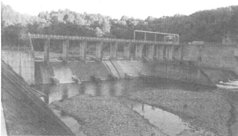
The Poutu intake on the Tongariro River.
