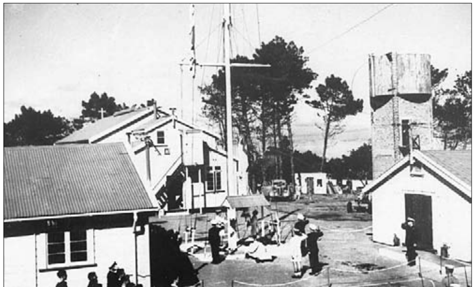
Figure A1.1. Water tower, Motuihe Island, near Auckland, c. 1950, showing structure with original doors, windows, and brickwork intact (held on file at Auckland Conservancy, DOC).
