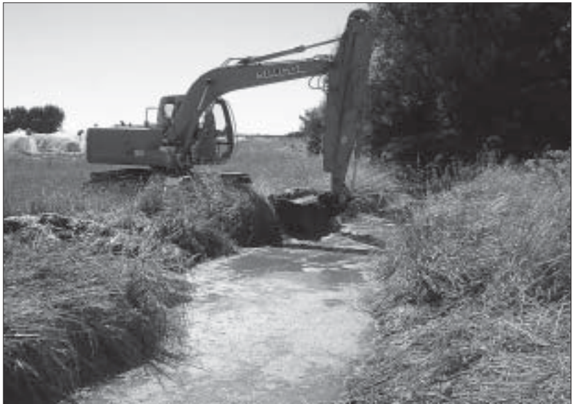
Figure 3. Mechanical clearance in Foothills Drain using an excavator.
