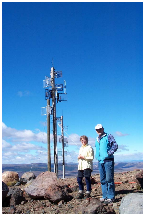
Site visit by board members to Tukino, Tongariro National Park – Vodaphone/Genesis communications installation to the left.
