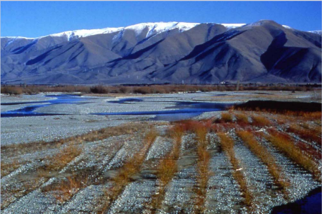
River engineering works - willow plantings
