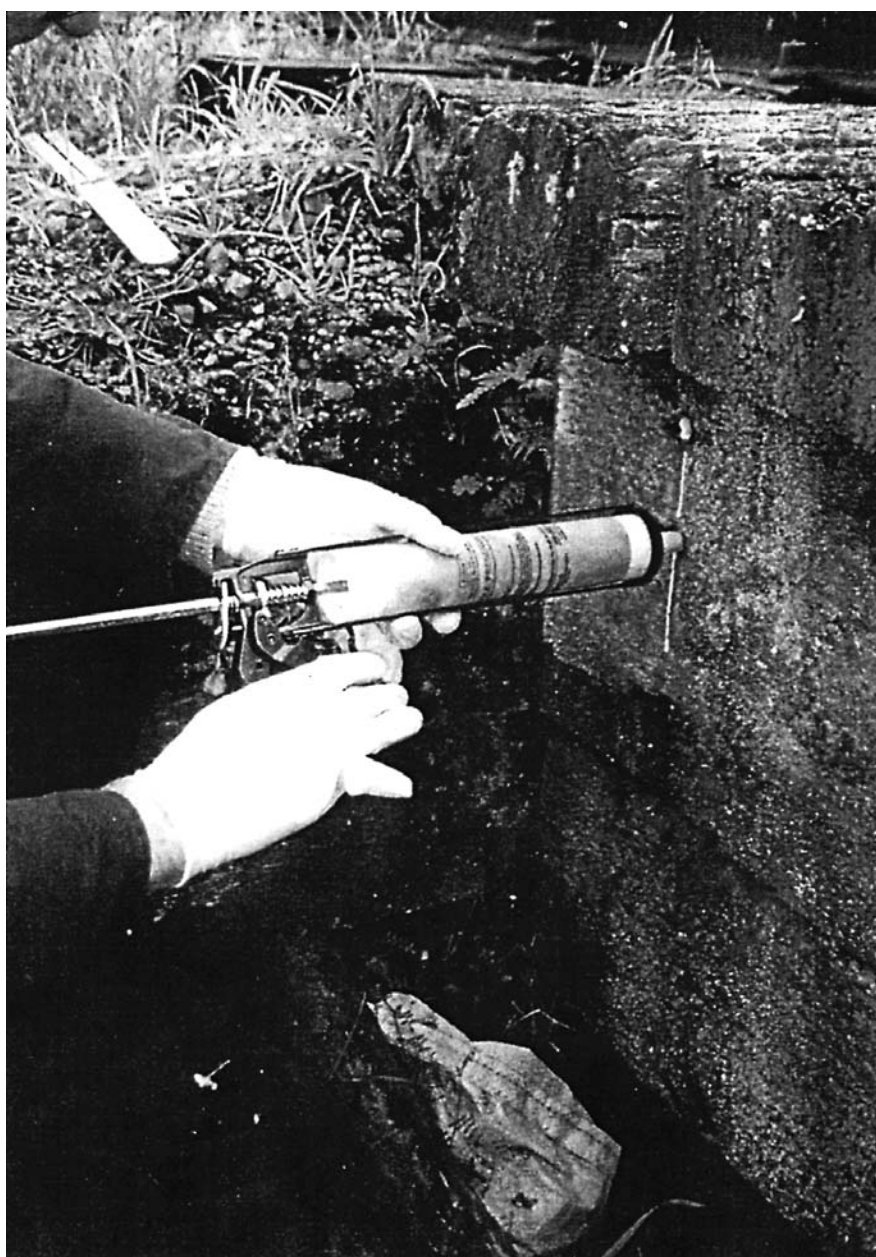
Fig. 18: Injecting Polegel with a caulking gun.
