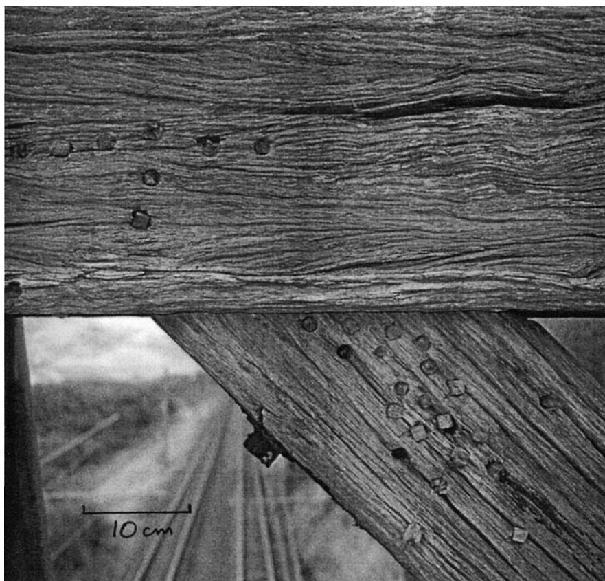
Fig. 5: Top chord and strut of a simple Howe truss, showing old inspection holes, some without hardwood plugs. Pukerua Bay road bridge over NIMT.
