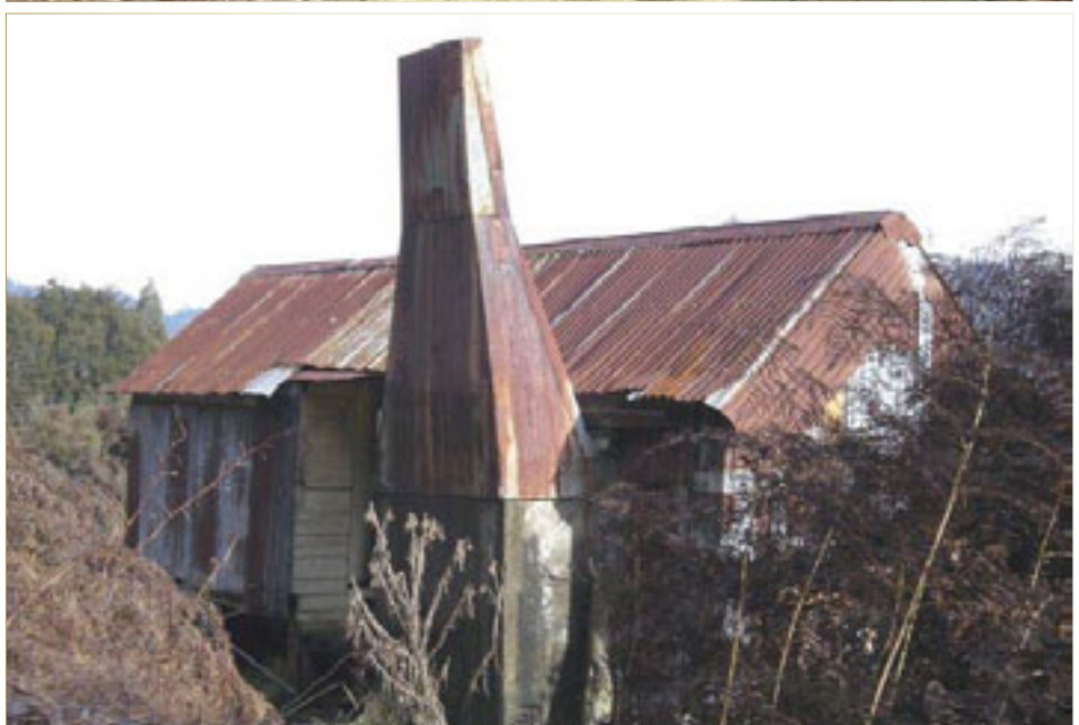
Photo 24: Rangers Hut, rear view, looking south west. J. BREEN DOC 2005.
