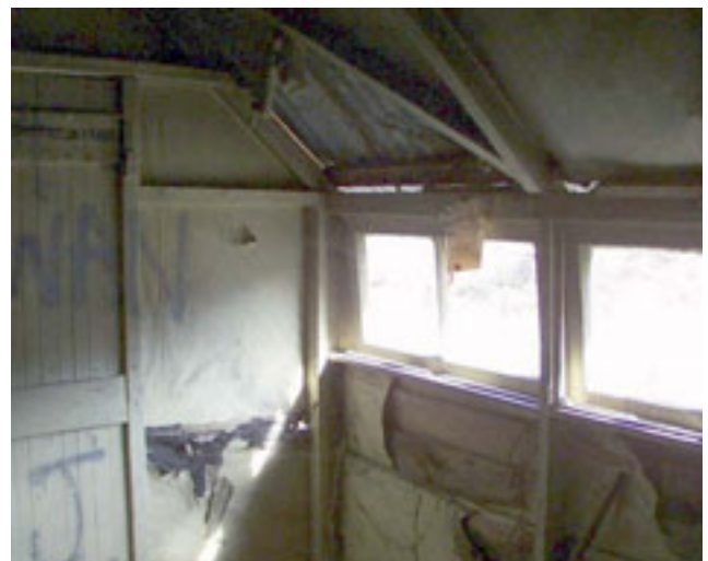
Photo 28: Interior view of the middle room, looking south. J. Breen, DOC, 2005..
