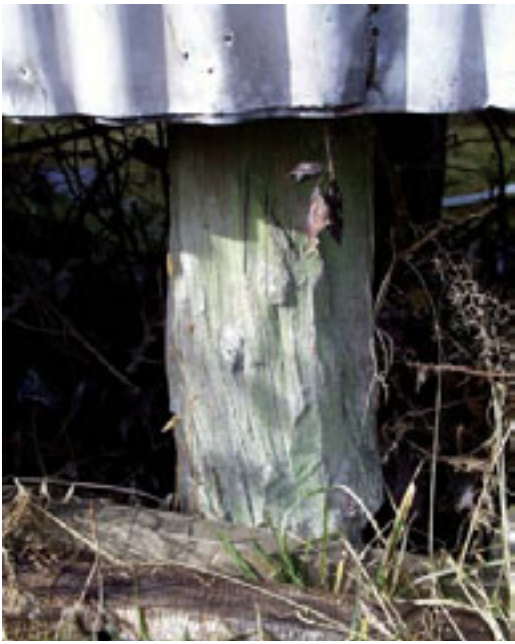
Photo 18: Detail of a pile cut from the bush. J. BREEN, DOC, 2005.
