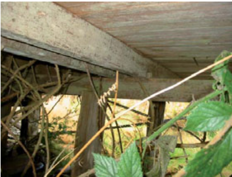
Photo 19: Detail of sub floor framing, south room. J. BREEN, DOC, 2005.
