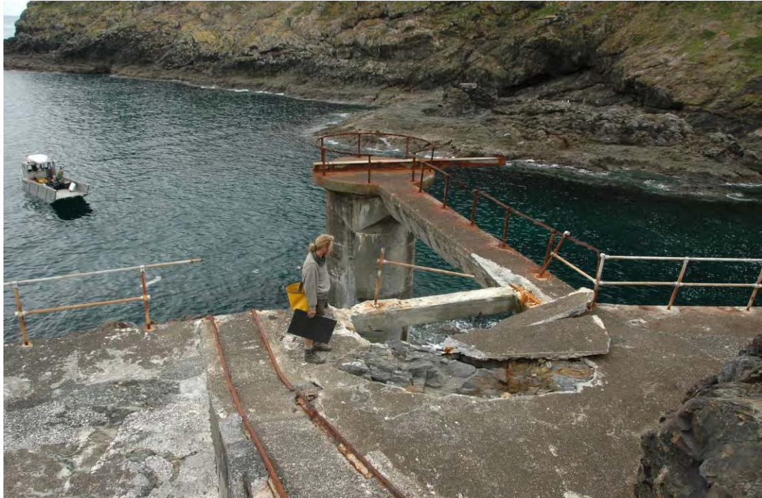
Figure 159 – The landing being inspected by Ranger Grant Oakes after the storms of 2008.
