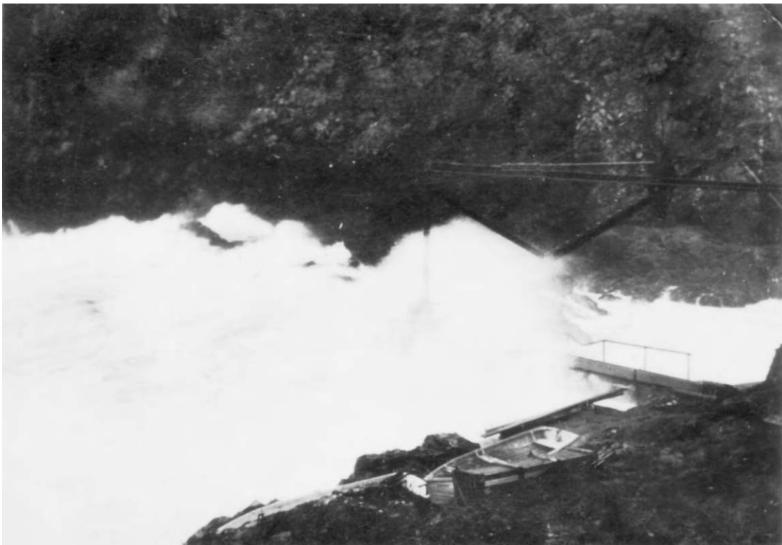
Figure 155 - The landing during a 1940s storm, note the dinghy lashed down.
