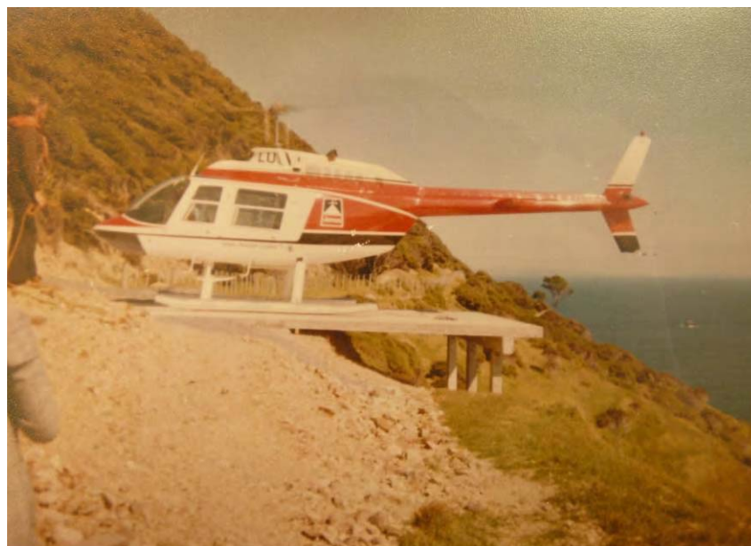
Figure 147 - The new helipad, 1970s.
