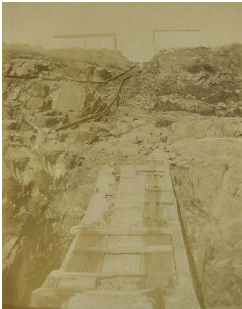
Figure 158 – Damage done to the tramway after a particularly rough storm, June 1943.
