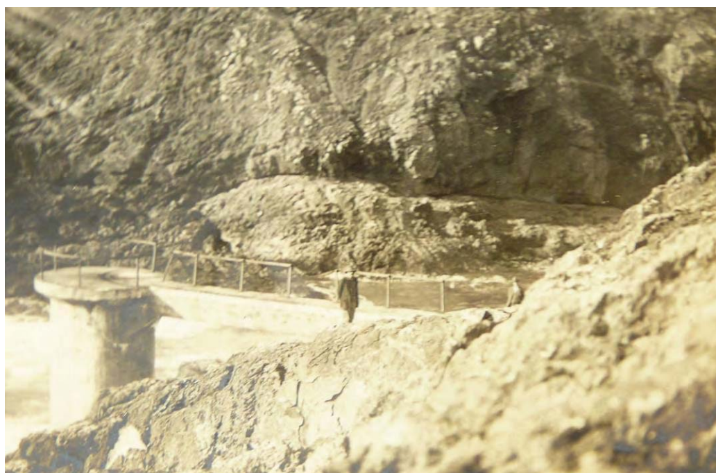
Figure 157 – The landing after a storm had washed the crane away, August 1924.
