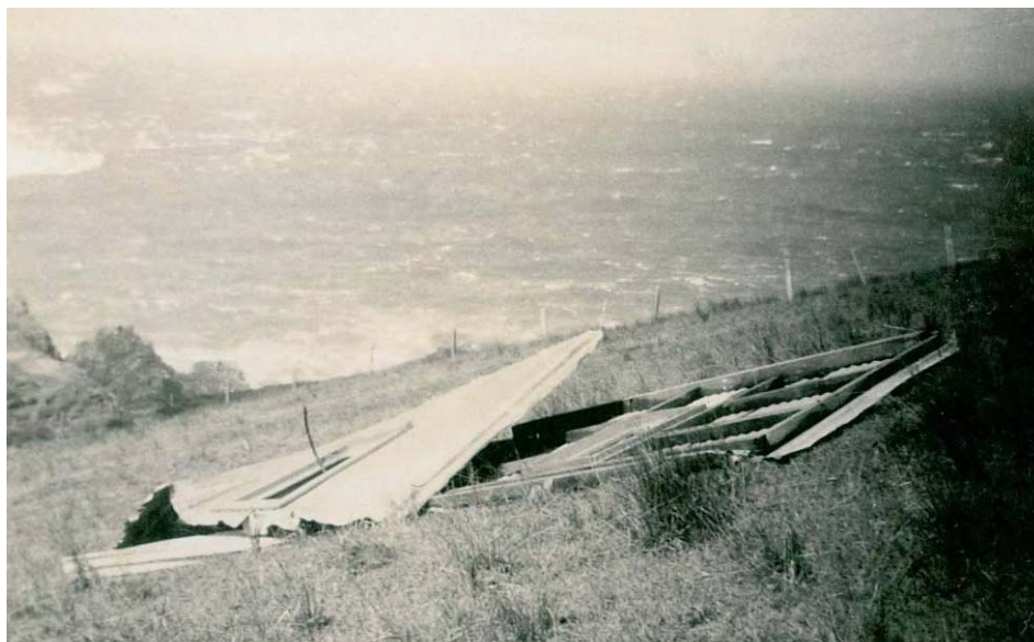
Figure 156 - One of the fowl houses after a storm, 1940s.
