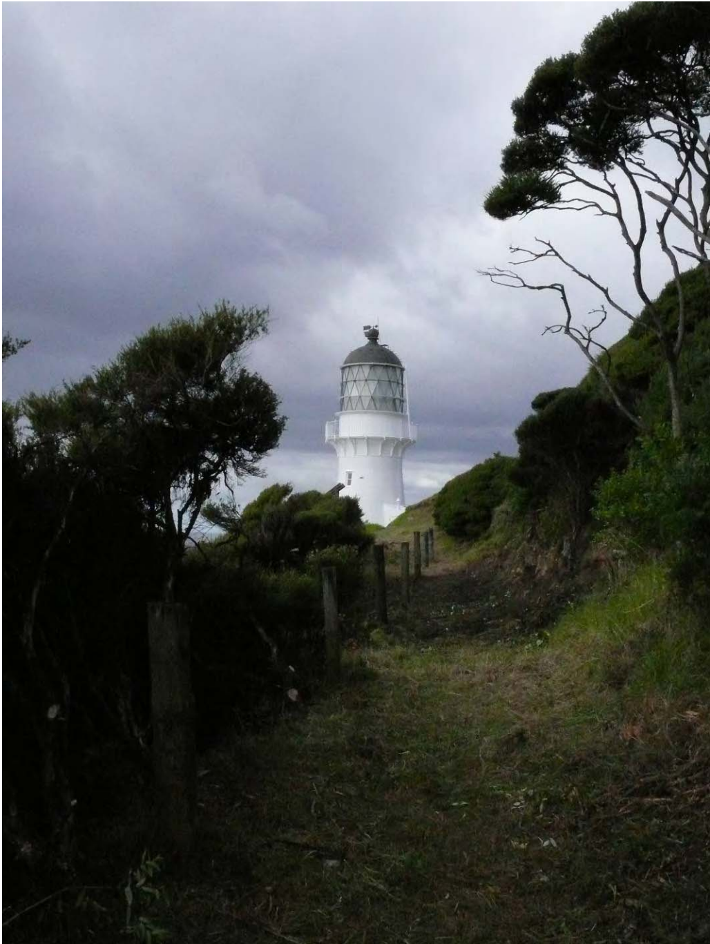
Figure 197 – A cleared portion of track, 2008.
