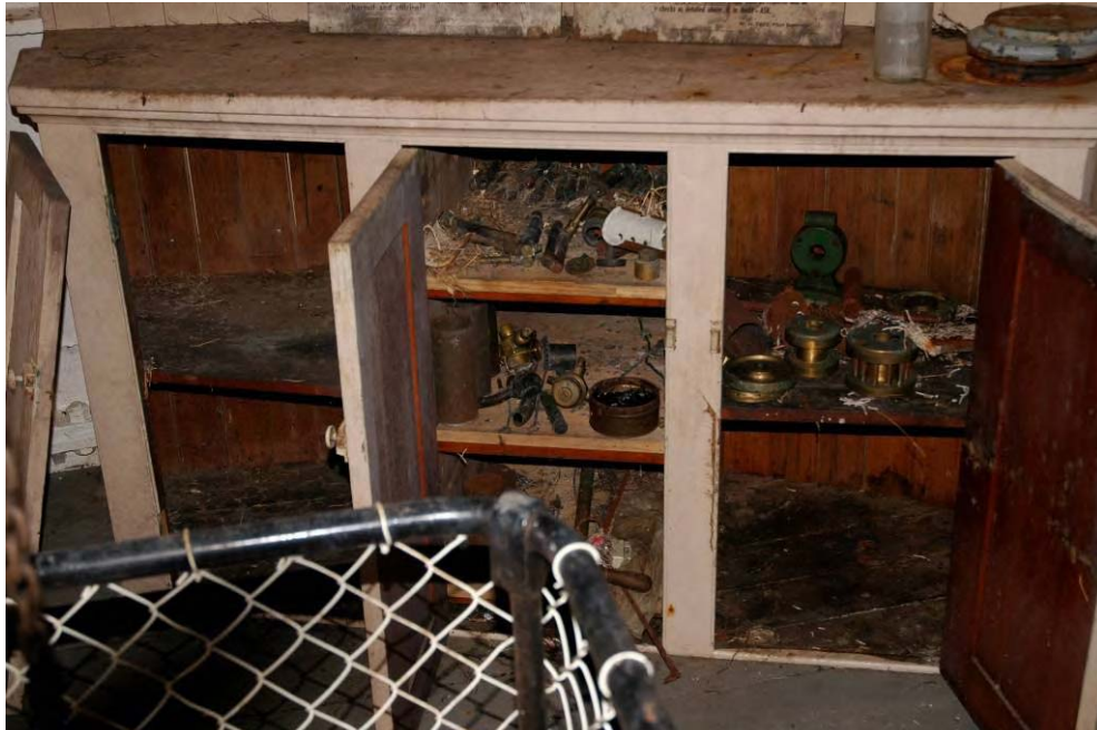
Figure 193 – The spares cupboard on the second floor of the lighthouse before cleaning, 2007.
