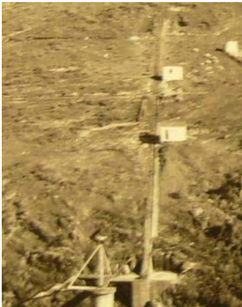
Figure 87 – The stores shed and engine shed on tramway during replacement of boat shed.
