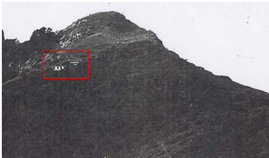
Figure 92 - The pump house.
