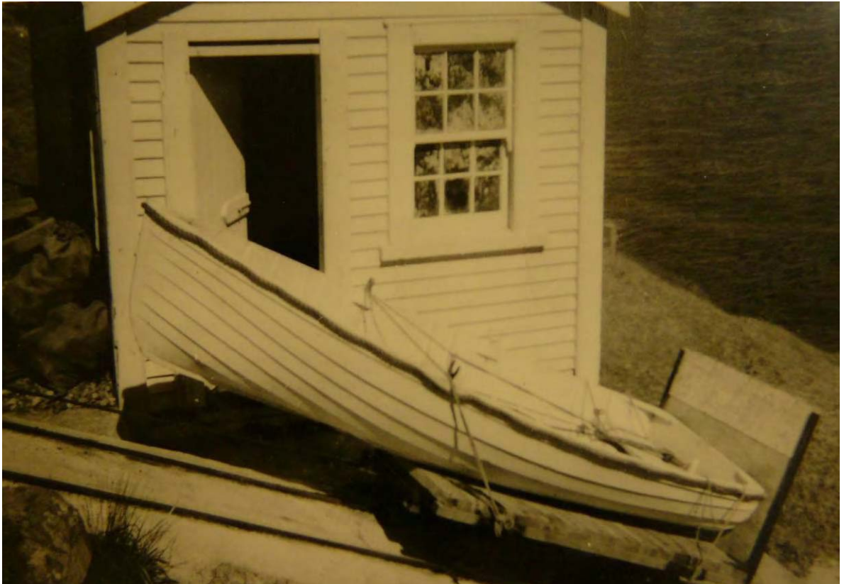
Figure 84 – The stores shed behind the boat that is being winched up the tramway.
