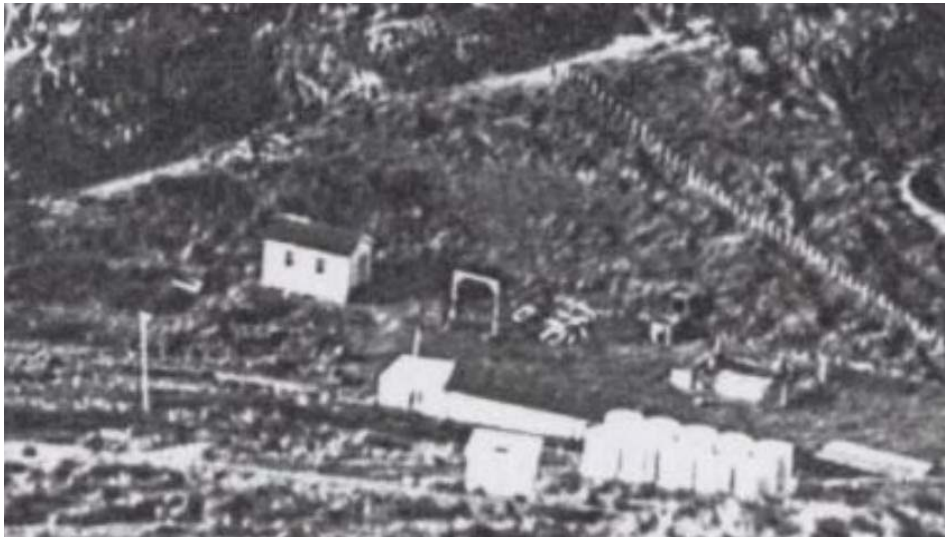
Figure 90 - The workshop after the forge's demolition.
