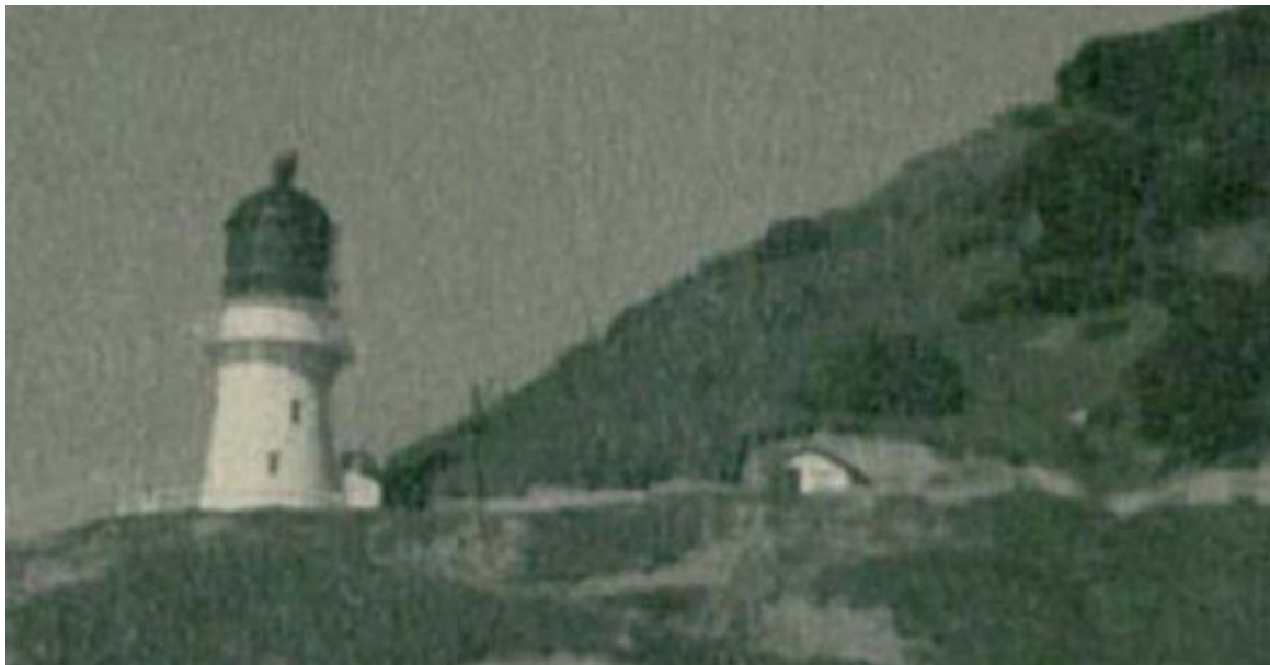
Figure 76 – The kerosene store located to the right of the tower.
