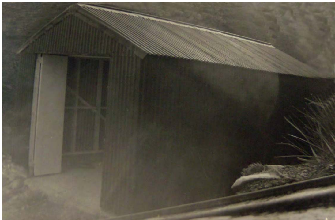
Figure 83 – The exterior after construction (and before being painted).
