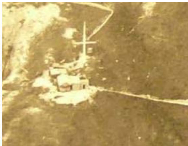
Figure 66 – The signal hut after modifications.
