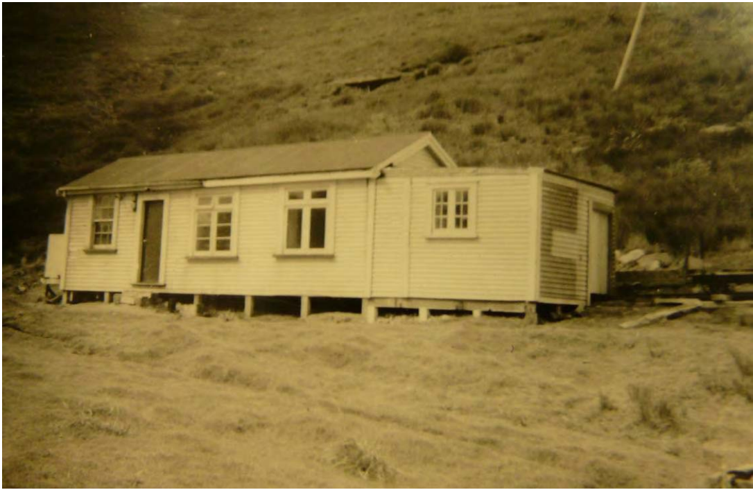
Figure 60 – The schoolhouse after the addition of the extra room.
