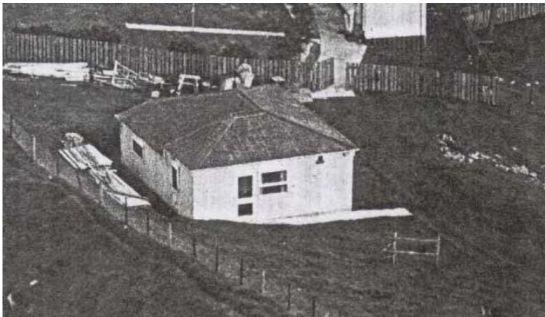
Figure 74 – View of the power house from the northwest.
