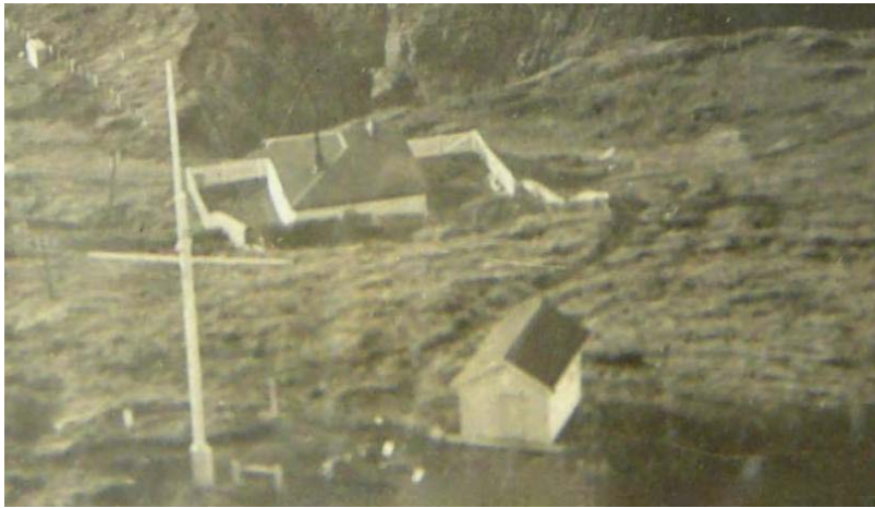
Figure 65 – The signal hut reverse view before modifications.
