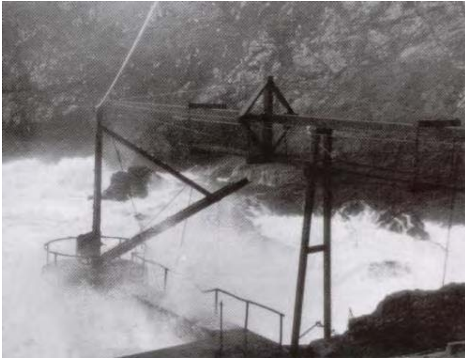
Figure 37 – The crane during a storm with the barriers removed.
